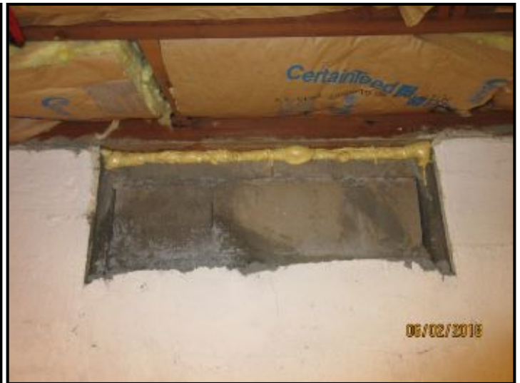
Basement window opening infilled during 2007 renovation/expansion.
