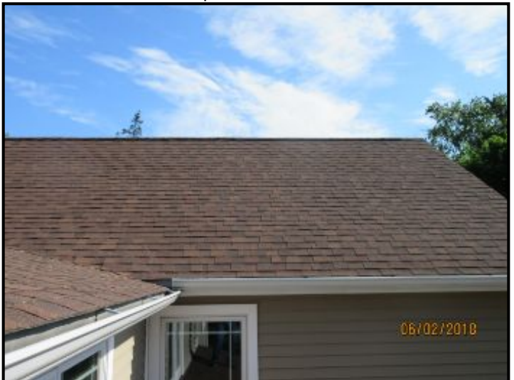
Upper roof in good condition.
