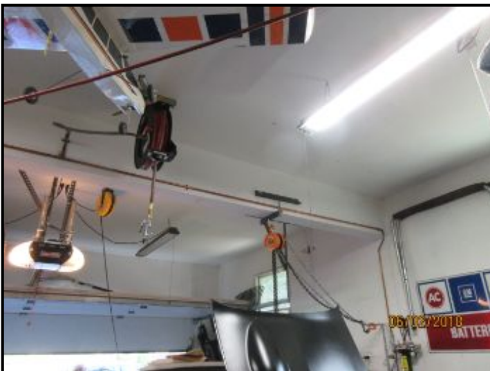
Limited review due to finished ceilings and walls.
