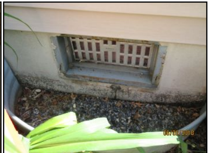
Screened vents noted at foundation walls.
