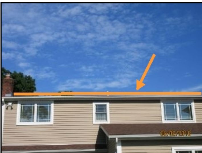
Roof ridge beams appeared straight and even.
