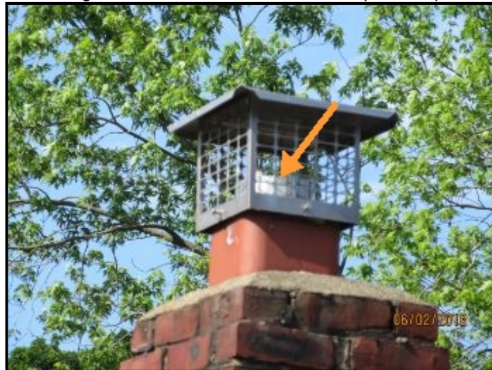
Metal chimney liner observed.
