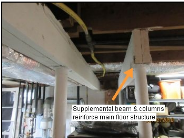
Floor Structure: 9x5 Wood main beam supported by steel lally columns, Supplemental beam and columns noted.
