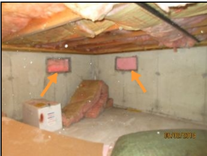
Screened vents noted at foundation walls.
