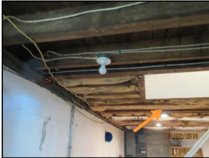
The main floor (above play area) was insulated with fiberglass batts.
