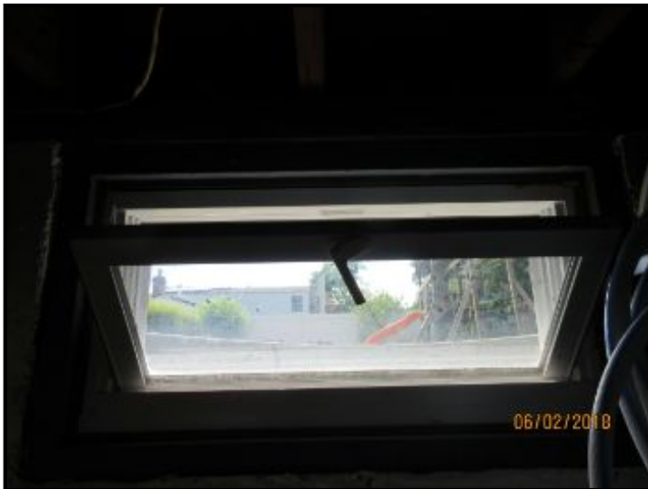
Vinyl framed Hopper windows noted. Operated windows appeared functional.
