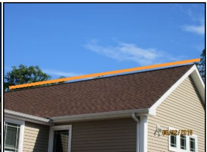
Roof ridge beams appeared straight and even.
