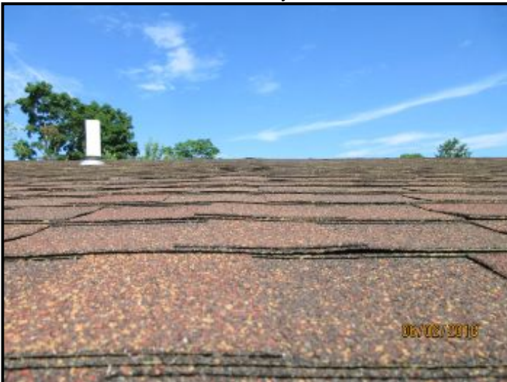
House top asphalt roof covering appeared to be approximately 11 yrs old.
