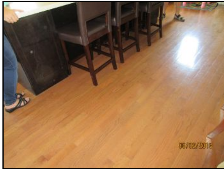
Engineered hardwood flooring noted
