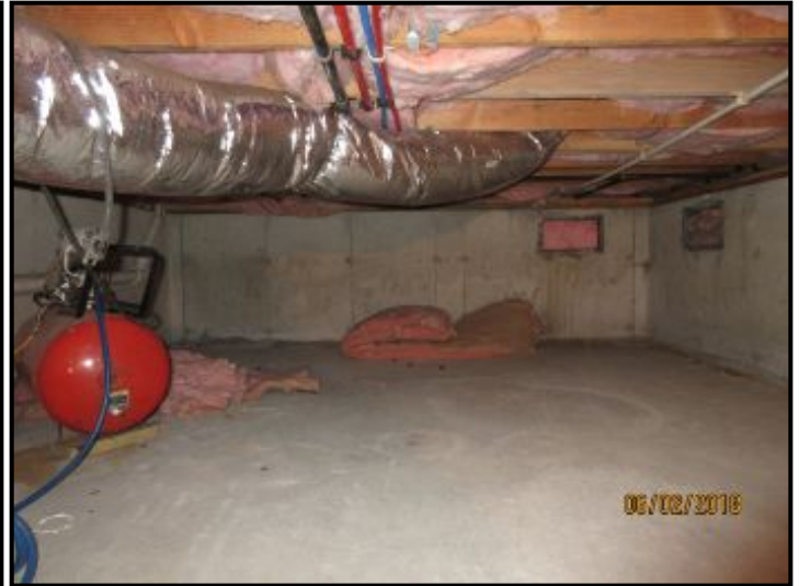
Crawlspace floor is concrete. Dampness: None observed
