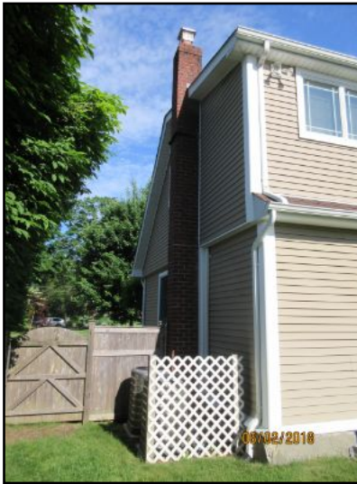
EXTERIOR Southeast Exterior
