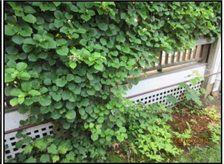
LIMITATION: Limited review due to a lack of access to deck structure beneath.
