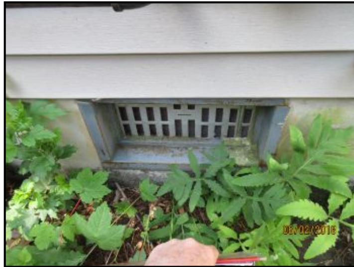
Screened vents noted at foundation walls.
