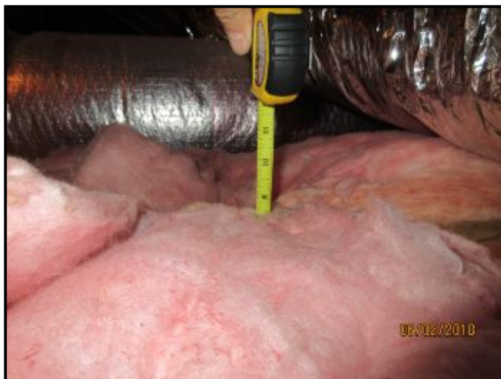
Insulation depth varies 9+ inches (R-31 overall); Good Insulation.
