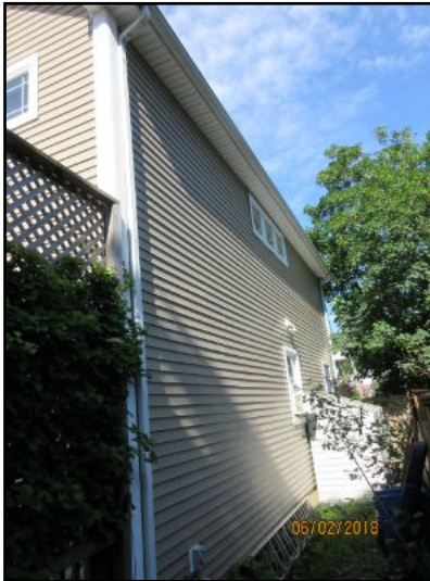
EXTERIOR North Exterior
