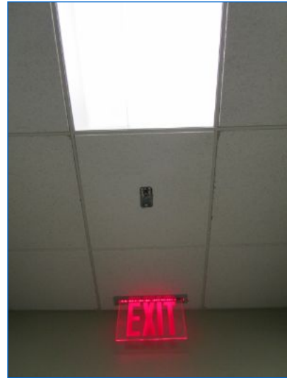
Exit signs noted for egress.
