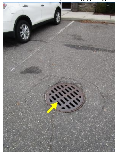
Storm drain located beyond the paved area above the parking garage.
