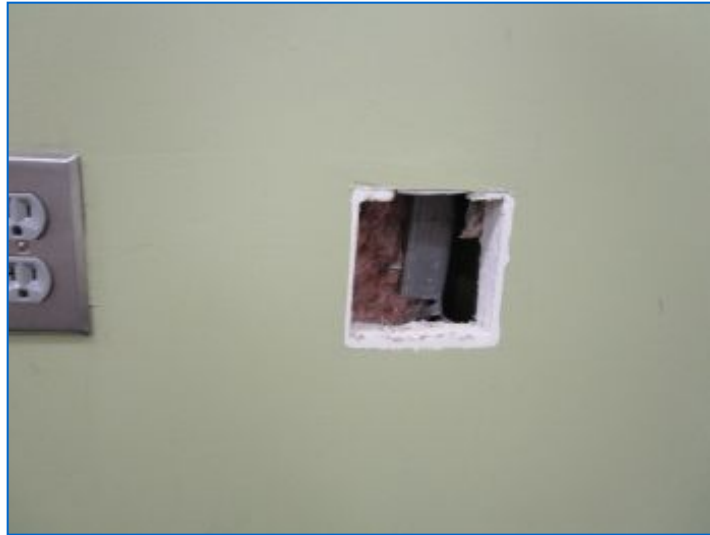
Apparent electrical box removed.
