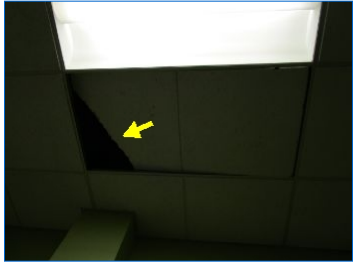
Some cosmetic damages were observed at ceiling tiles.
