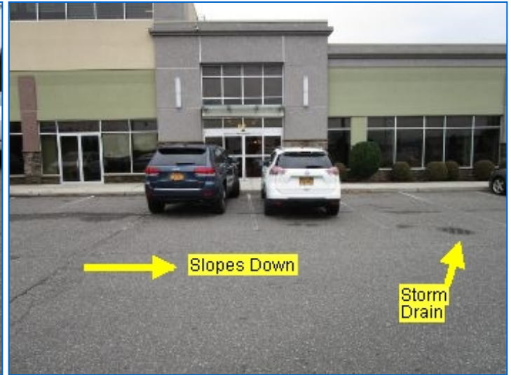
Shows location of storm drain located beyond the paved area above the parking garage.
