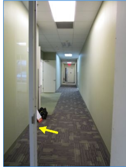
Hallway (rear portion); self-closing fire door/s noted.
