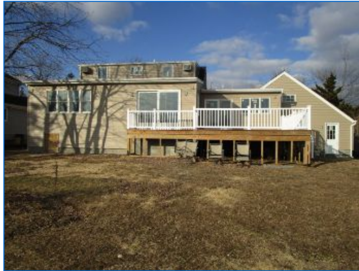
EXTERIOR East Exterior
