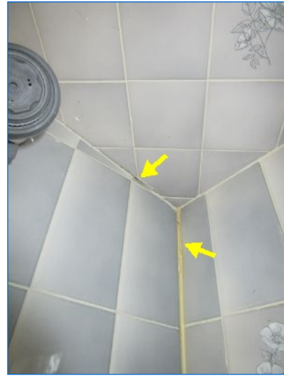
Cracked grout at corner joints noted to have been caused by the structure elevation. Grout repairs recommended to prevent water entry.
