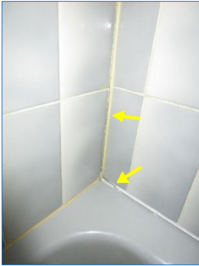
Cracked grout at corner joints noted to have been caused by the structure elevation. Grout repairs recommended to prevent water entry.
