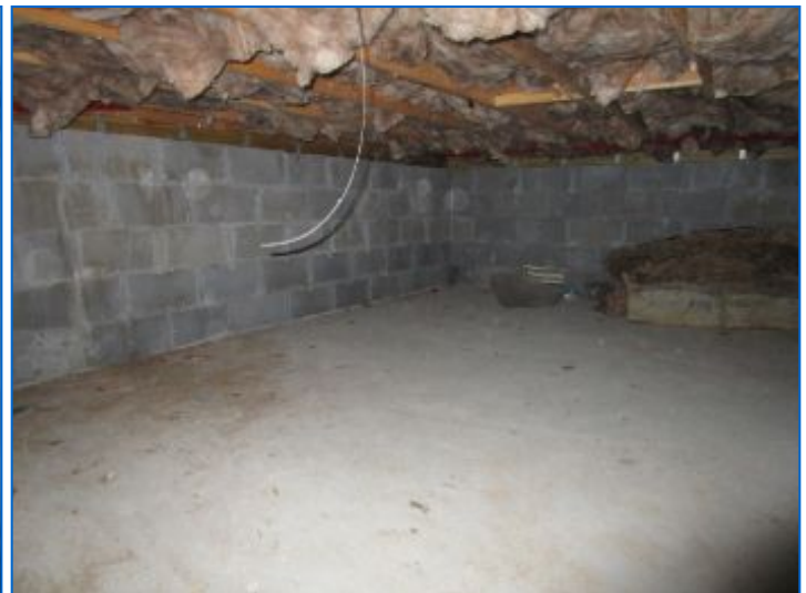
East crawlspace area, looking north.
