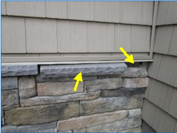
Missing and loose cap stones at front wall; incomplete work.
