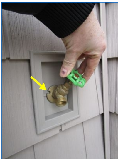
Hose bibs were not properly mounted; twisted occurs at PEX tube connection when used causing potential for leak inside the wall. Recommend completing installation of hose bibs asap to prevent the twisting.
