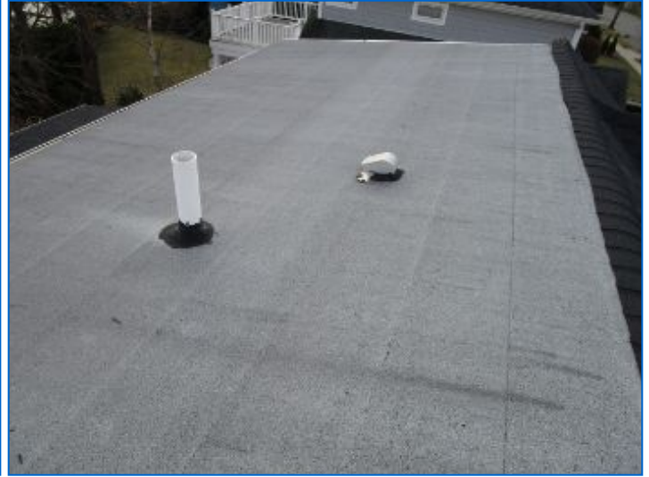
Asphalt rolled roofing noted for low-slope roof area.
