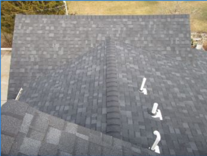
The roof had one layer of asphalt shingles installed at the time of the inspection.
