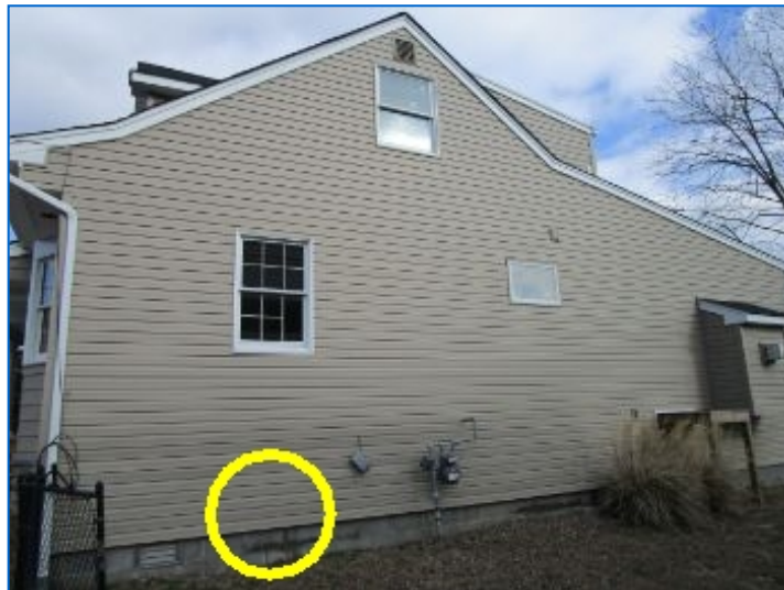
EXTERIOR South Exterior
