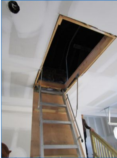
Pull-down ladder located in Garage.
