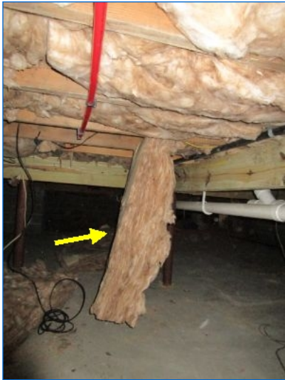
Batt insulation was observed to be hanging/missing at a few joist cavity locations. Recommend restoring missing/hanging insulation and securing in place using insulation support wires.
