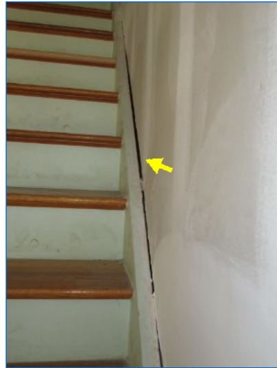
Molding and finishes not yet completed.
