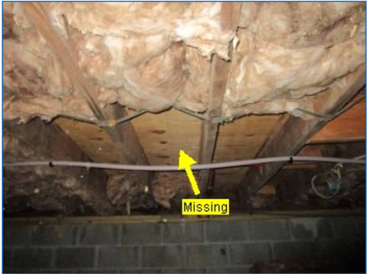
Batt insulation was observed to be hanging/missing at a few joist cavity locations. Recommend restoring missing/hanging insulation and securing in place using insulation support wires.
