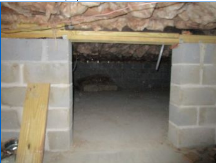
Interior access to east crawlspace area.
