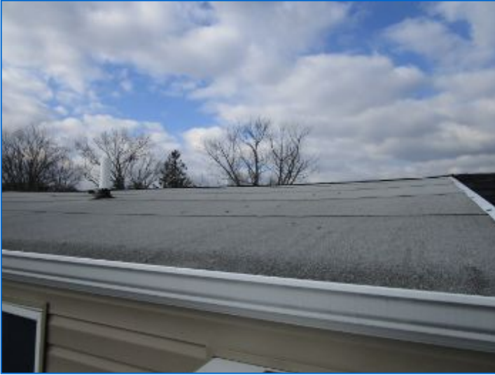
Asphalt rolled roofing noted.
