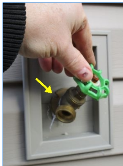
Hose bibs were not properly mounted; twisted occurs at PEX tube connection when used causing potential for leak inside the wall. Recommend completing installation of hose bibs asap to prevent the twisting.
