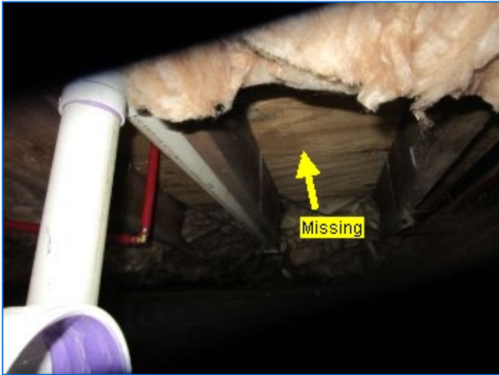
Batt insulation was observed to be hanging/missing at a few joist cavity locations. Recommend restoring missing/hanging insulation and securing in place using insulation support wires.
