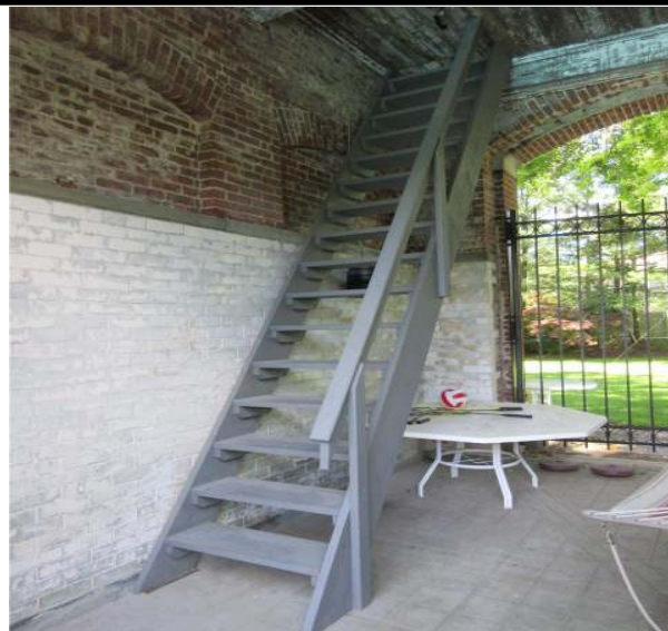
IMG_1181.JPG Stair to 2nd floor hatch with handrail in good condition.
