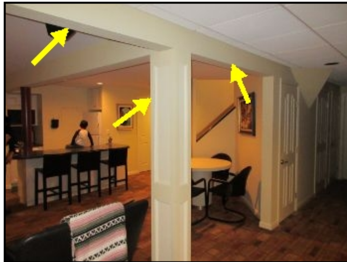
Main beam(s) and columns were Mostly finished/concealed; unable to fully inspect.
