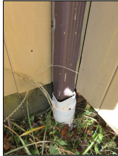
Most downspouts appear to drain to underground drywell.
