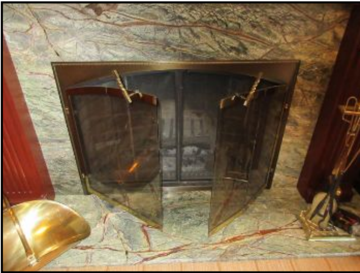
Wood burning fireplace in Den on Main level.
