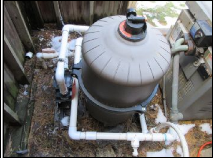
Pool filter appeared generally to be in serviceable condition at the time of the inspection, however was shut-down, winterized and could not be tested at time of inspection.
