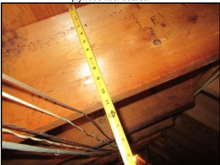
Roof Structure: 2x8 and 2x10 Rafters 16" O.C. w/collar-ties, 2x8 ridge beam, Plywood roof boards.
