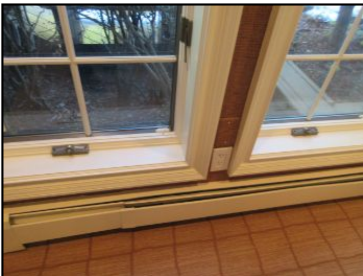
Wood framed Casement windows noted.
