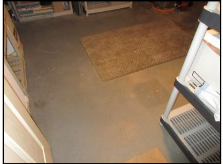
No evidence of moisture penetration was observed at the visible portions of the concrete floor slab at the time of inspection.
