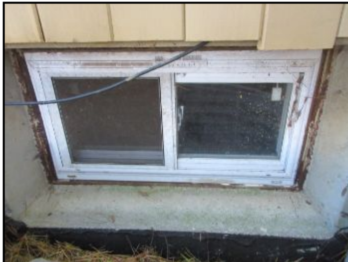
Insulated vinyl framed sliding windows noted.
