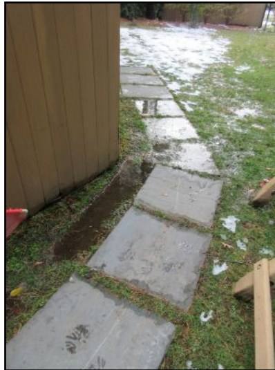
Puddling at northern side yard may be an indication of poor drainage here. Landscape drainage improvement may be considered such as below grade perforated drain piping with drywell.
