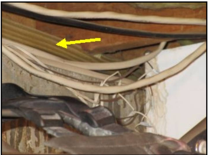
REPAIRS: Section of the Sill Plate at east side was replaced with pressure treated wood. Past termite water damage is suspected.
