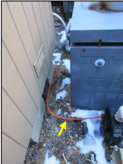
New fuel line from new above ground oil tank.
