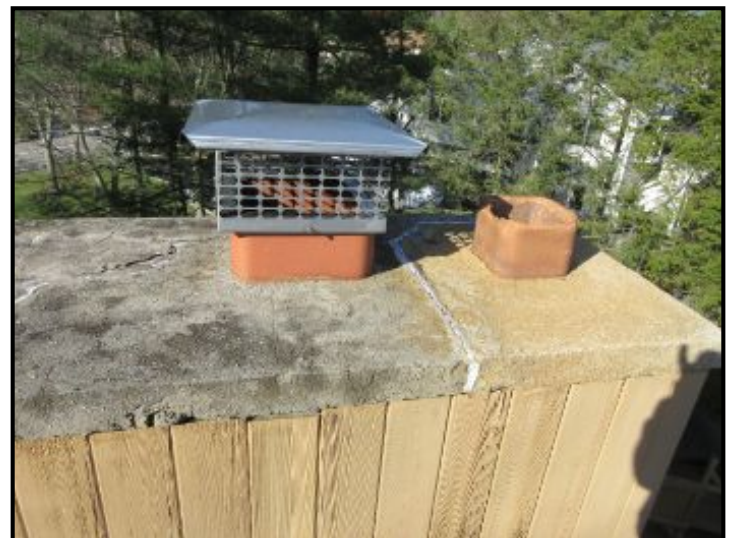
Combined fireplace and furnace chimney brick enclosure noted.
