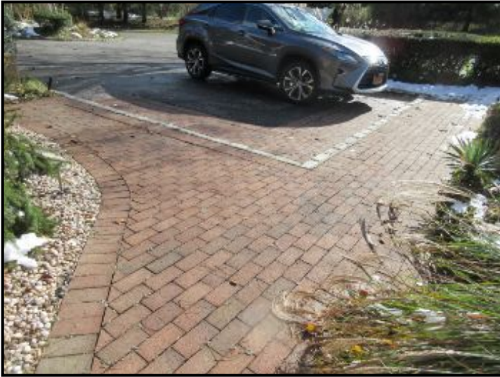
Brick walkways noted.
