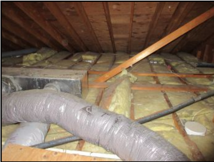
Installed in joist cavities.
