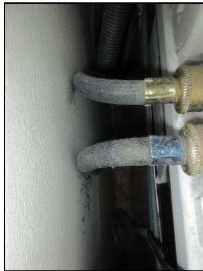
Leaks: No signs observed at time of inspection.
