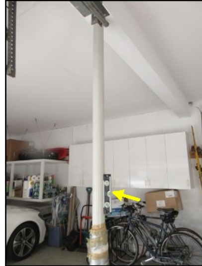
Limitation: Garage structure was Largely concealed by finishing systems; unable to fully inspect.
