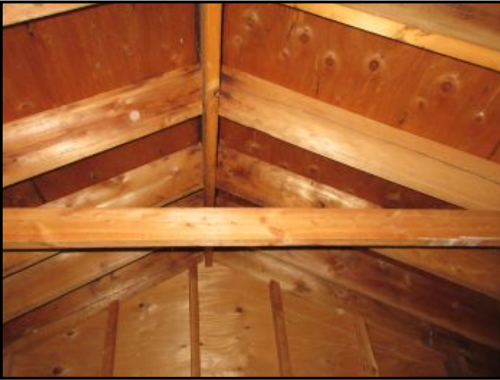
Structure at northern end.
