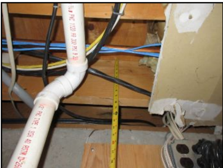
Main Floor Structure: 5x12 wood main beam supported by steel lally columns, 2x10 Joists 16" O.C. (w/cross braces), plywood floor boards.
