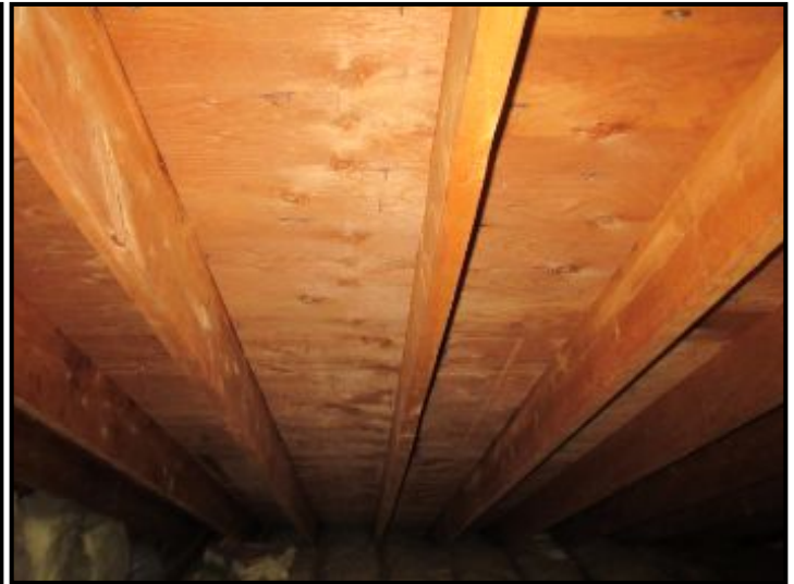
Roof structure in generally sound condition.
