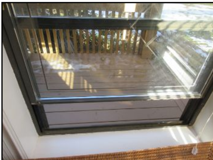
Aluminum framed Double Hung windows noted; original windows (30 yrs old).
