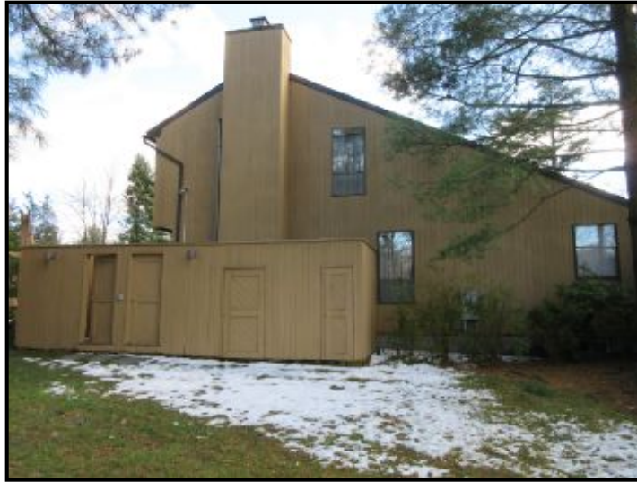
EXTERIOR North Exterior
