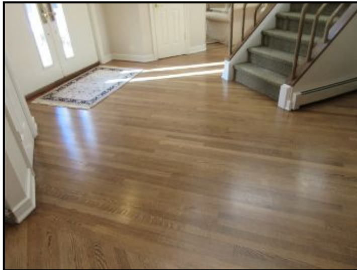
Hardwood flooring noted throughout 1st floor in good condition.
