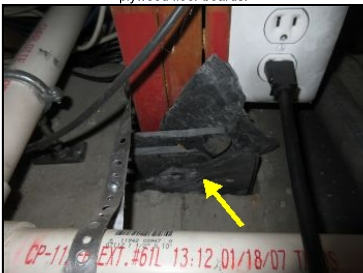
Main Floor Structure: 5x12 wood main beam shimmed at foundation wall; slate shims.
