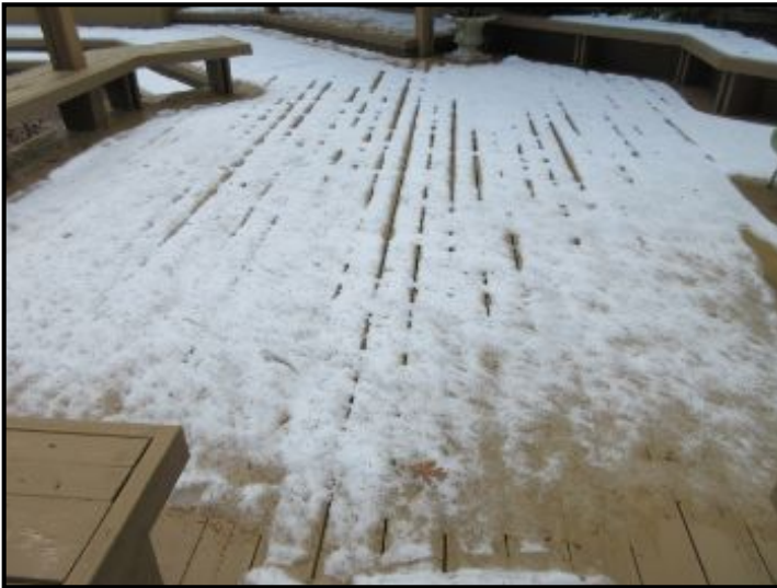
Limited inspection: Areas of the deck planking was covered with snow at the time of inspection. unable to fully inspect.
