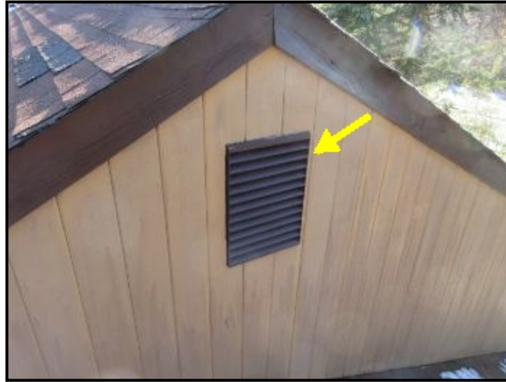
Gable-end louver vent(s) noted for attic ventilation.
