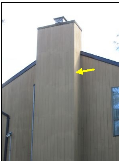
Architectural chase noted
