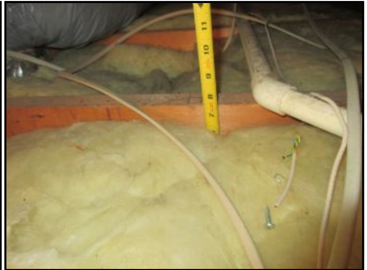
Insulation depth varies 6 - 8 inches (R-24 overall). NOTE: Latest energy conservation standards call for 9-10 inches (R-30). Additional insulation may be installed where possible for enhanced energy efficiency of the home.
