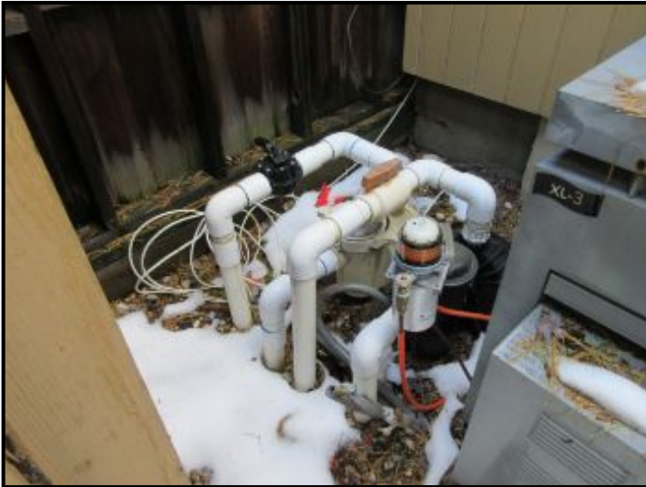
No apparent cracks that would cause leakage in the PVC piping, however piping was drained at time of inspection.
