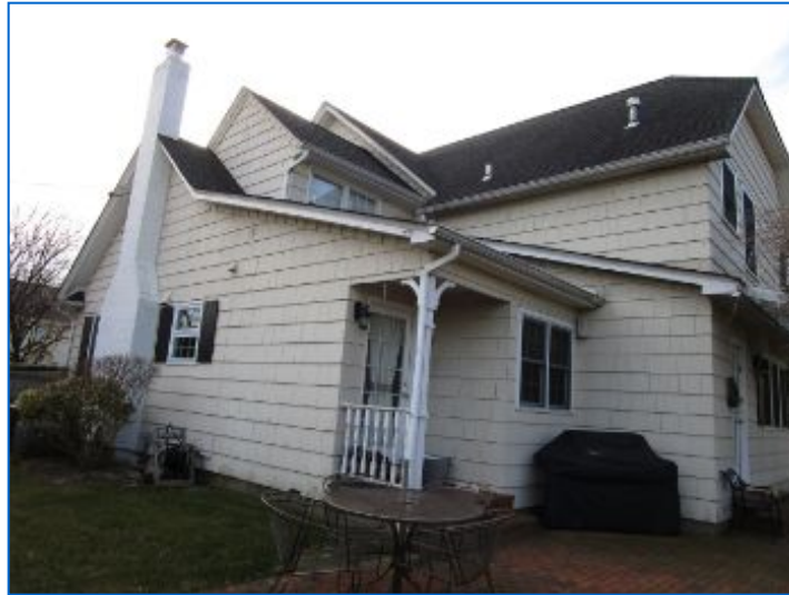
EXTERIOR North Exterior
