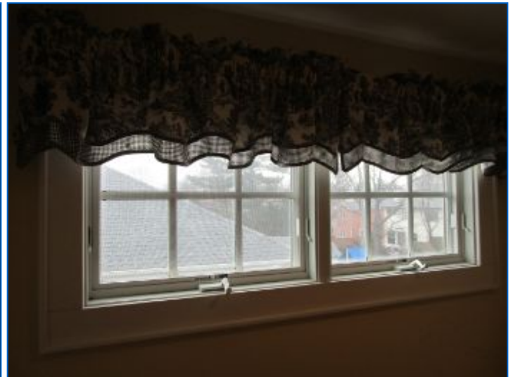
Casement windows noted in attic.
