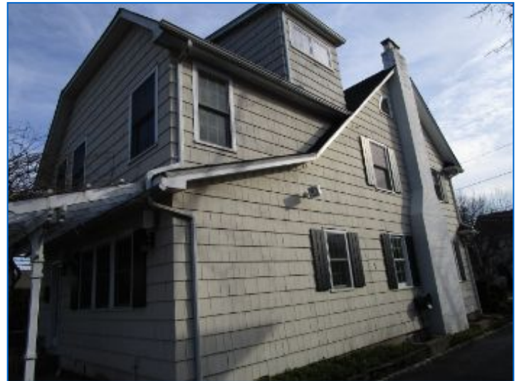
EXTERIOR South Exterior
