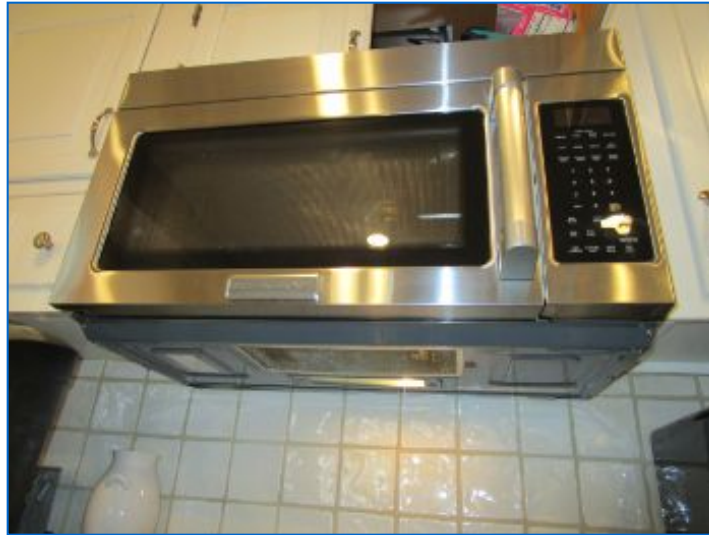
Microwave had an operable Exterior vented type vent fan with filter and light.
