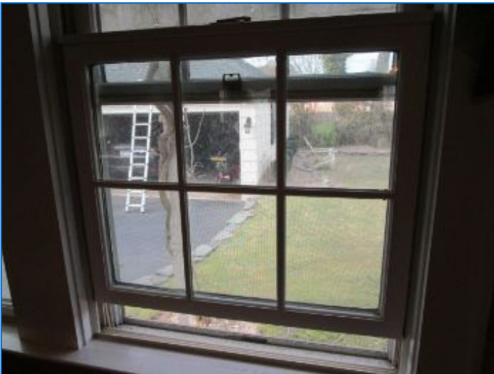
Most windows in the home were double-hung wood framed windows.
