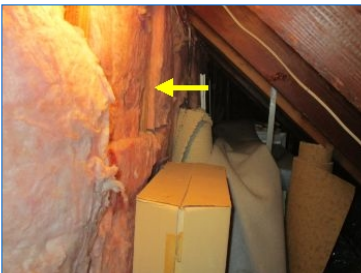
Insulation installed in knee wall cavities.
