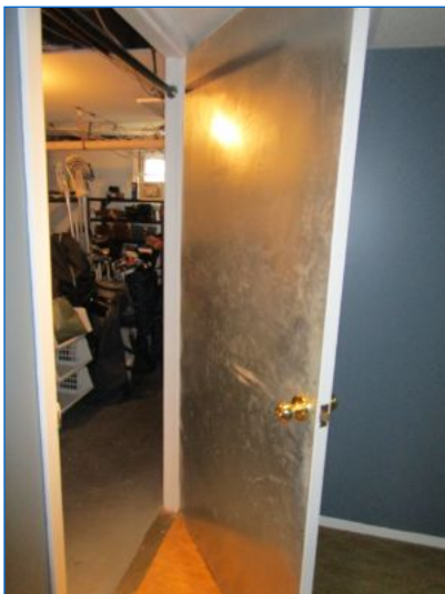
Boiler room door with sheet metal cover on interior noted.
