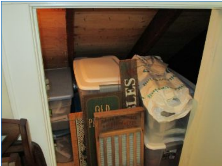
Moderate storage was noted in the attic eave spaces at time of inspection.
