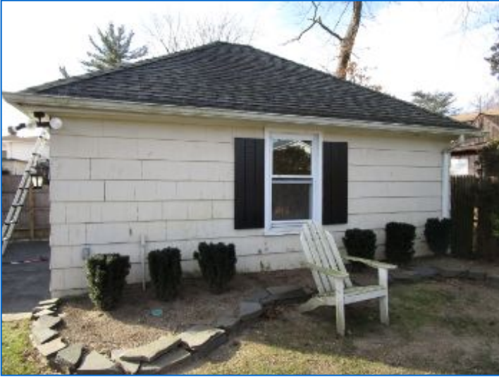
GARAGE General Conditions
