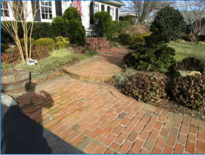
Walkways: No major system safety or function concerns noted at time of inspection.
