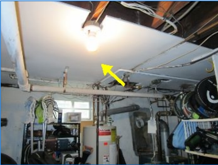
Boiler room ceiling was largely covered.
