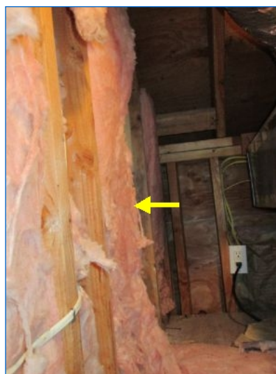
Insulation installed in knee wall cavities.
