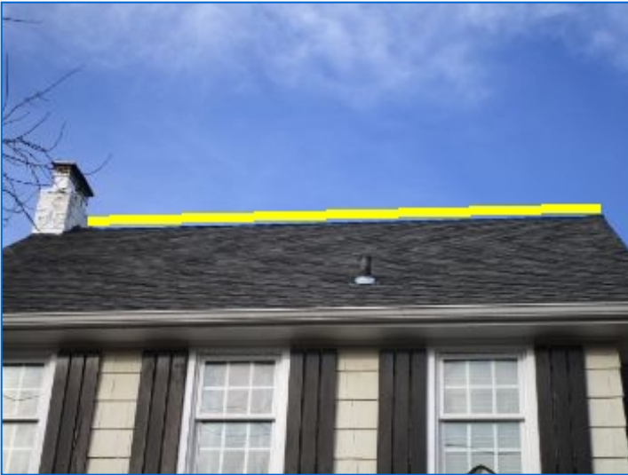
Roof ridge beam appeared straight and even.
