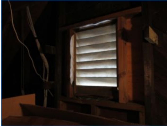
Attic (unfinished spaces) appeared to be adequately ventilated.
