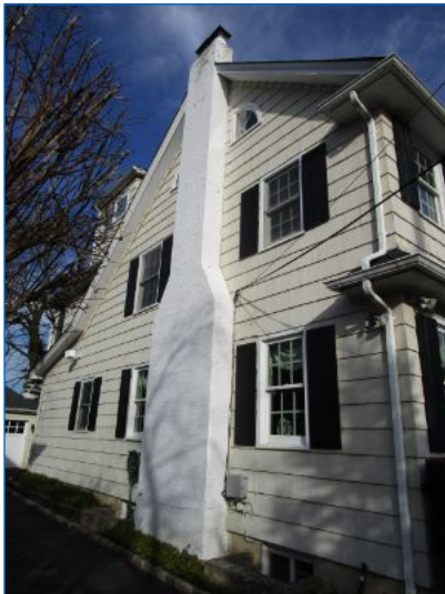
EXTERIOR South Exterior
