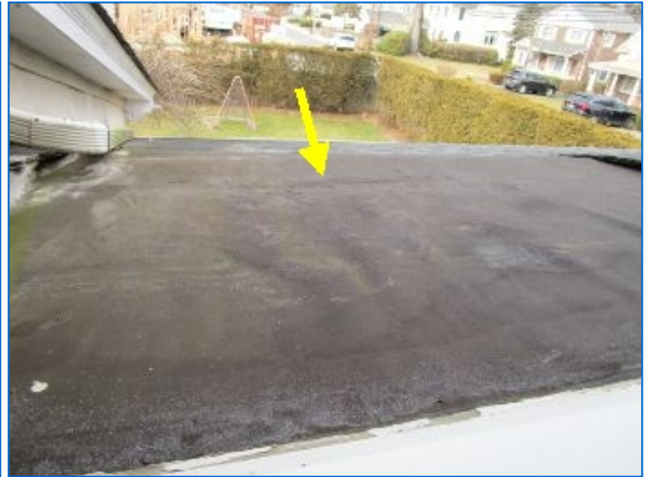
Semi-flat roof, rubber membrane noted here.
