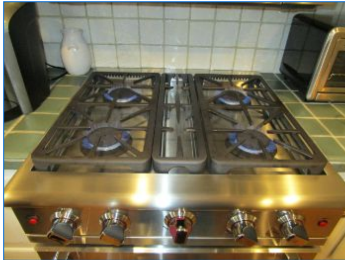
Gas-fired range; operable. Range appeared to be approximately 1 yrs old.
