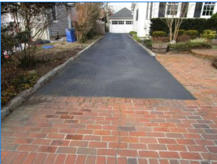
Maintenance: Asphalt driveways require sealing every 3-5 yrs to prevent water penetration and freeze-thaw damage.
