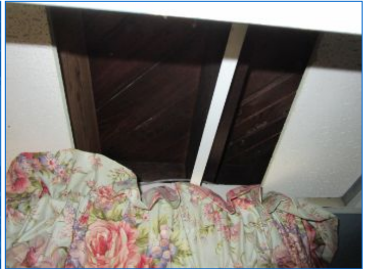
Main floor structure accessed through hung ceiling in basement office.
