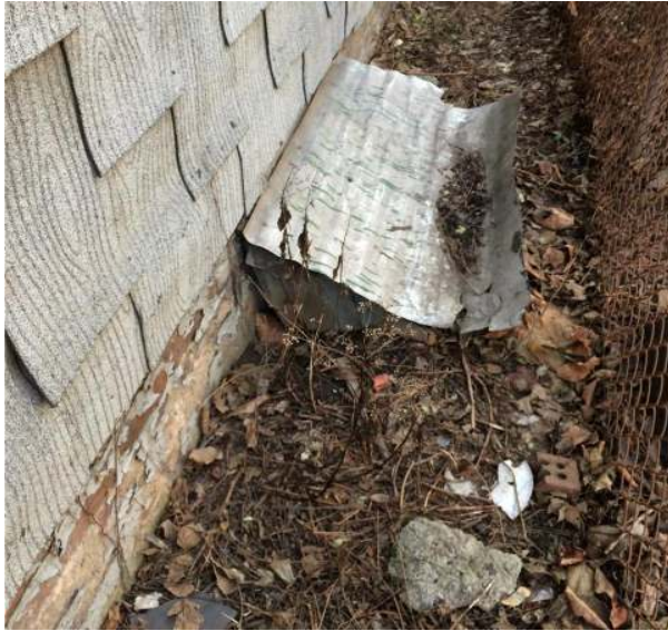
IMG_0891.JPG Sheet metal access cover at side of house (unknown).
