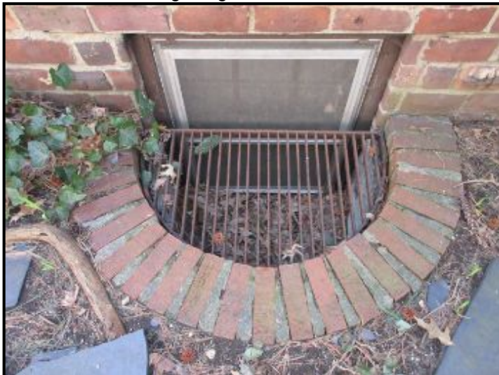
Masonry window wells with steel grating noted.
