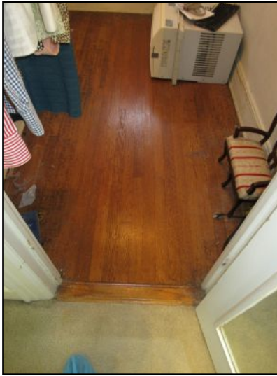
Hardwood floors beneath carpeting on 2nd floor.
