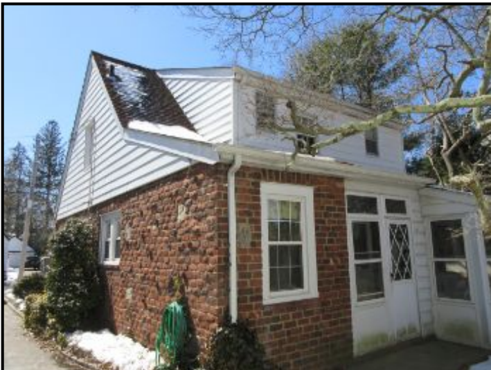
EXTERIOR North exterior
