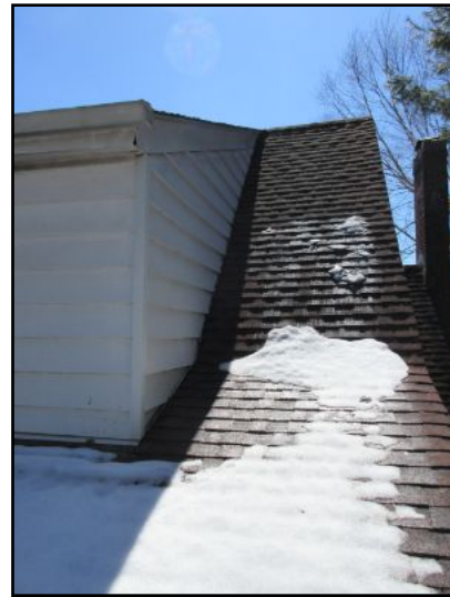
Partially snow covered, not fully inspected.
