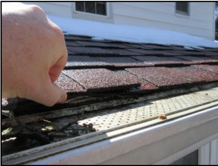
One layer of asphalt shingles noted.
