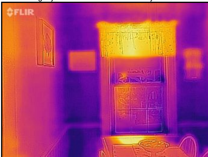
Dining room east wall is representative of the exterior wall insulation in the home. Typical insulation here is 3 inches thick, estimated at 9.5. This may be improved only slightly due to the limited wall cavity of 3.5". This may be improved only slightly due to the limited wall cavity of 3.5".
