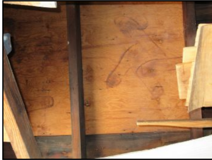
Roof board repairs noted.
