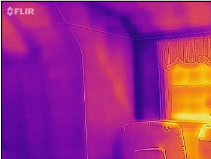
West bedroom southeast wall represents the average thermal condition for the home. Typical insulation here is 3 inches thick, estimated at R-9.5. This may be improved only slightly due to the limited wall cavity of 3.5".
