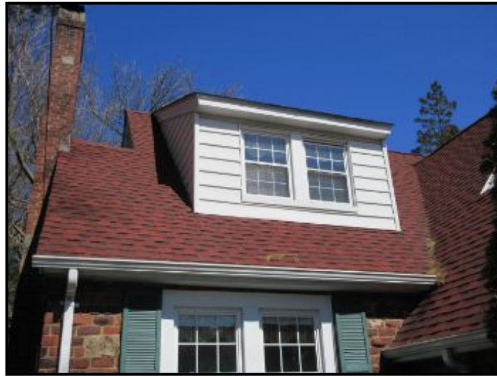
EXTERIOR South exterior
