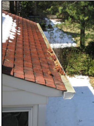
No major system safety or function concerns noted for the visible portions of the roof.
