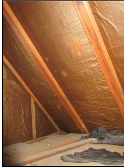
Fiberglass batts with kraft paper facing noted.
