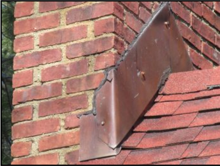
Copper flashing visible around chimney.
