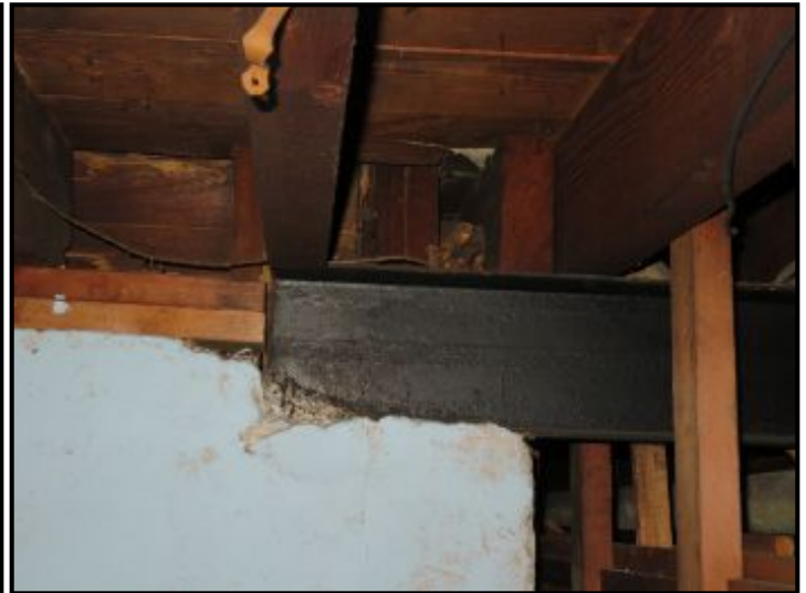
Floor Structure: Steel girder supported by foundation wall and steel lally columns, 3x8 Joists 16" O.C. (w/cross braces), T&G floor boards
