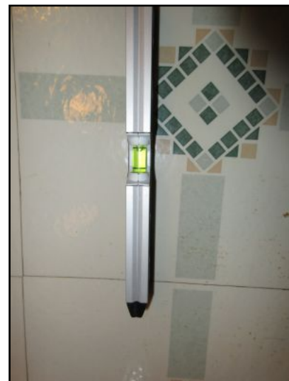
Bathroom floor pitched downward to shower base.
