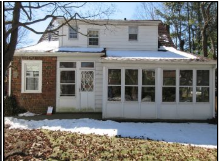
EXTERIOR North exterior
