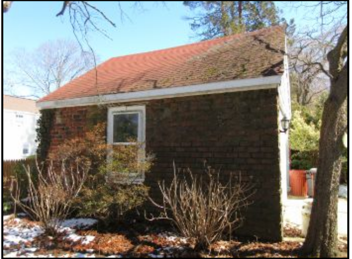
GARAGE Garage General
