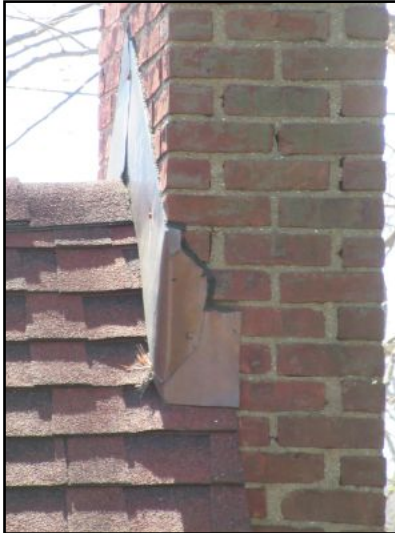
Chimney flashing appear intact and functional.
