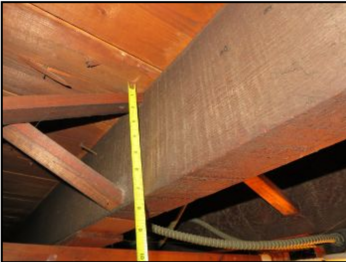
3x8 Joists 16" O.C. (w/cross braces), T&G floor boards
