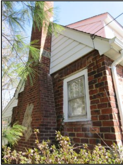
EXTERIOR West exterior
