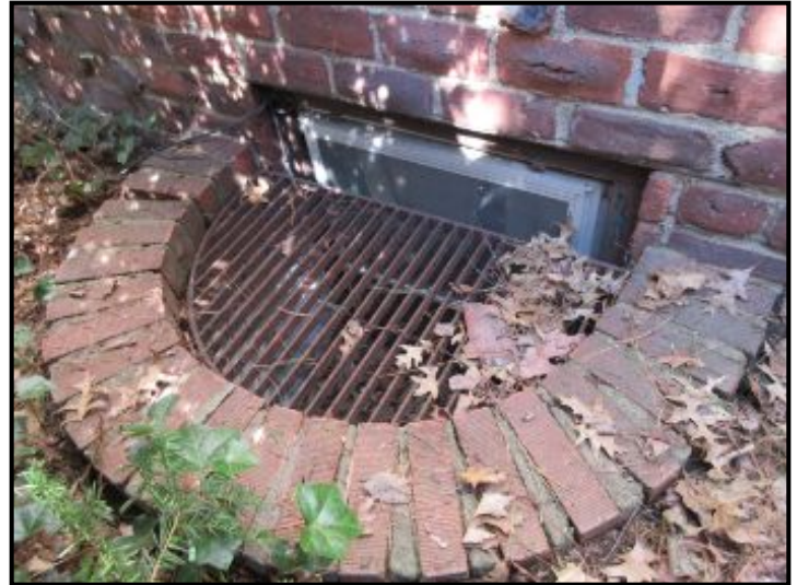
Masonry window wells with steel grating noted.
