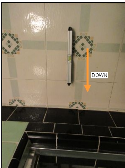
Bathroom floor pitched downward to shower base.
