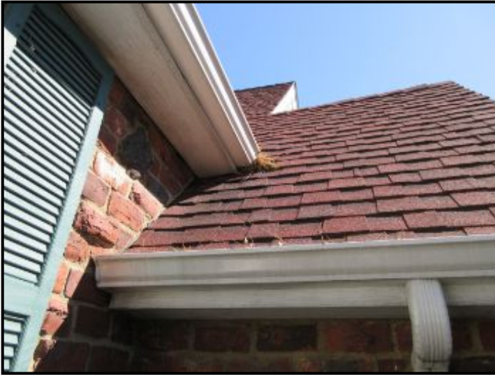
House top asphalt roof covering appeared to be approximately 8-10 yrs old.
