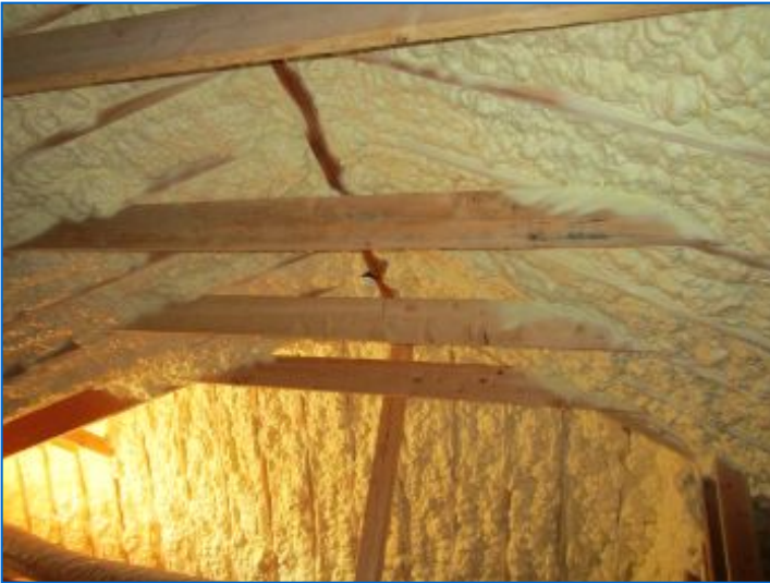
Insulation installed in rafter cavities / exterior wall cavities.
