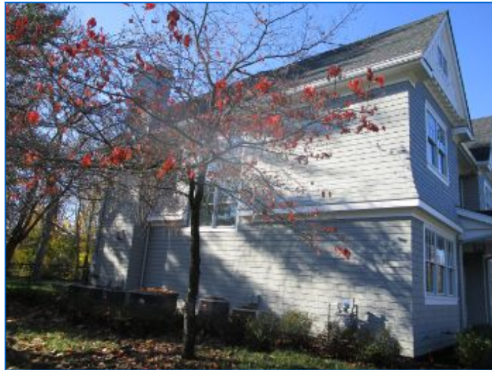
EXTERIOR East Exterior
