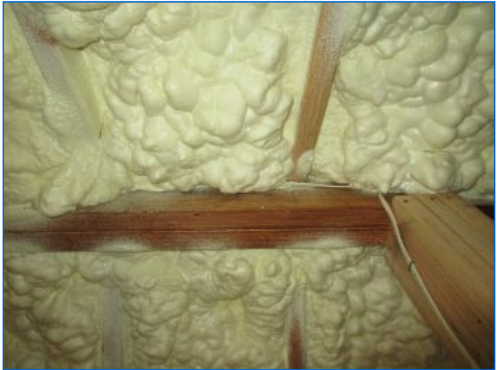
Insulation depth varied 10-11 inches (R-36 overall); Well Insulated.
