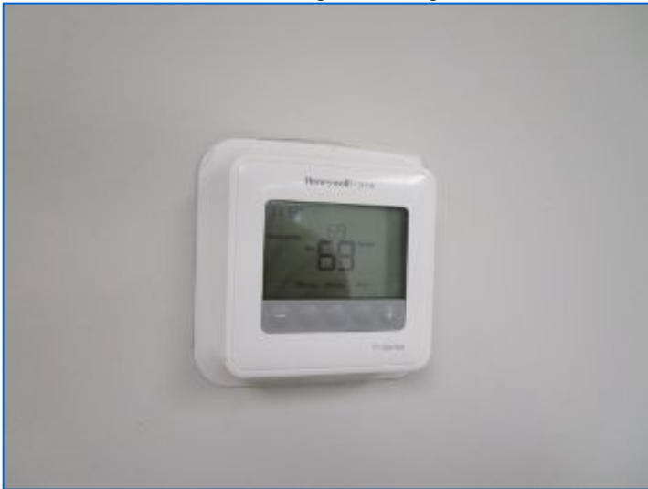
Digital Programmable type thermostat noted in Basement; for Heating & Cooling.
