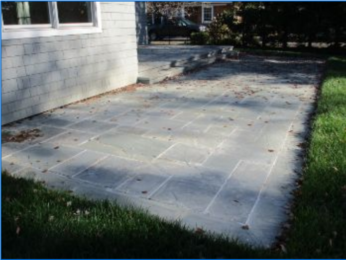
Patio: Bluestone in mortar noted.
