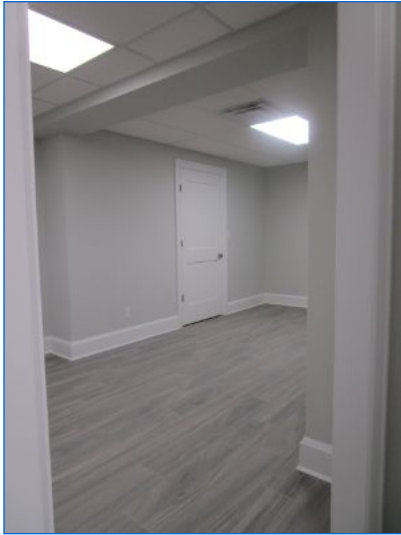
NE corner room.
