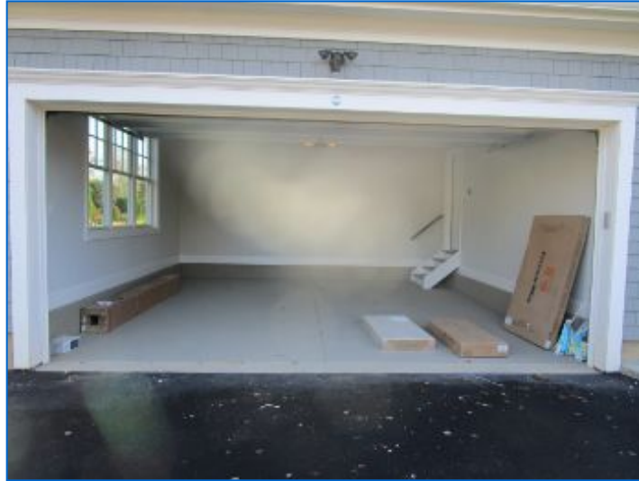
Garage structure is Integral to the house structure.
