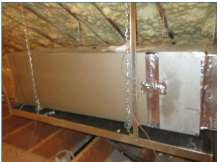
HVAC#3 ducted Air Handler located in the Attic serves the Maser bedroom suite.
