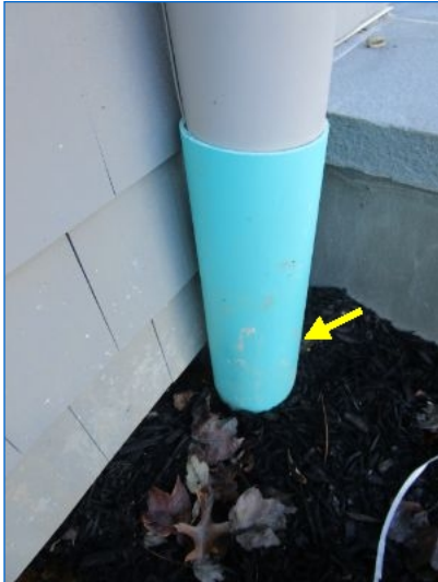
Downspouts apparently connected to underground drainage system; drywell. Downspouts apparently connected to underground drainage system; drywell.
