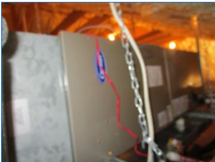
HVAC#3 ducted Air Handler located in the Attic serves the Maser bedroom suite.
