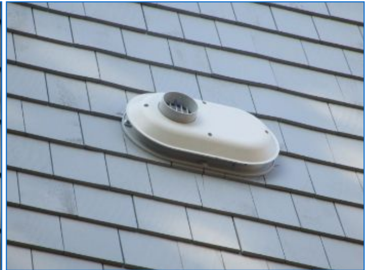
Boiler furnace vents noted at East exterior / mock chimney.
