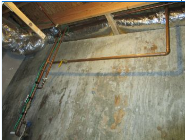
The home water supply pipes appeared to be properly bonded to the home electrical system at the time of the inspection.
