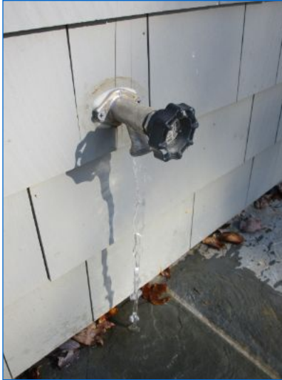
Hose bib at Rear was active at time of inspection.
