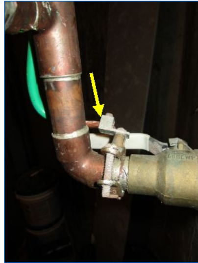
The home water supply pipes appeared to be properly bonded to the home electrical system at the time of the inspection.
