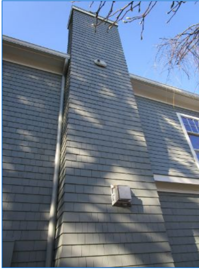
Chimney: Framed, covered with siding; apparent mock chimney.
