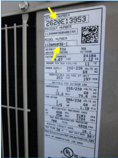
AC#1 Bryant Condenser data-plate/serial no. indicated a cooling capacity of 3 tons, and a manufacture date of 6/2020, (0.5 yr old).
