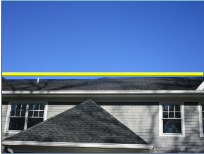
Roof ridge beam appeared straight and even overall.
