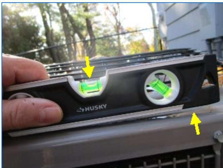
AC#2 Condenser was not level; this can shorten motor life. Suggest leveling mounting pad or the unit itself.
