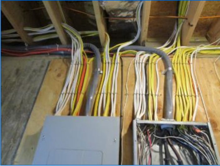
Distribution wiring observed consisted of copper, non-metallic sheathed cable.
