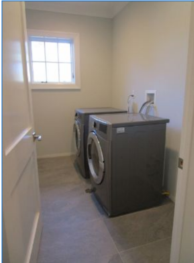
Laundry-1 Location: 2nd floor.
