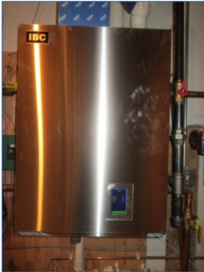
Boiler Type: Gas-fired, Tankless Hot Water Boiler combined with indirect storage tank domestic water heater; Manufactured by IBC.
