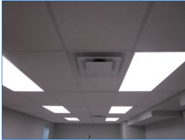
Acoustical tile w/grid ceilings noted.
