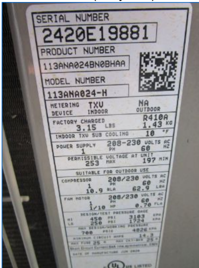
AC#3 Bryant Condenser data-plate/serial no. indicated a cooling capacity of 2 tons, and a manufacture date of 6/2020, (0.5 yr old).
