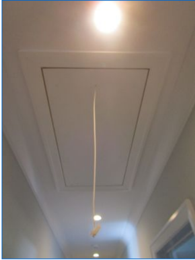
Pull-down ladder located in Hallway (2nd floor).
