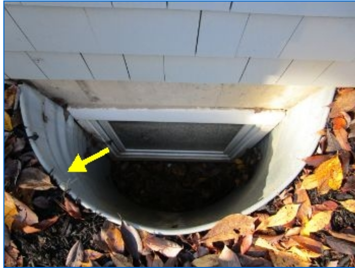
Steel window wells noted.
