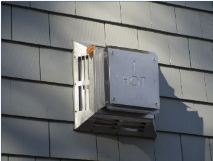
Gas fireplace direct vent noted at East exterior / mock chimney.
