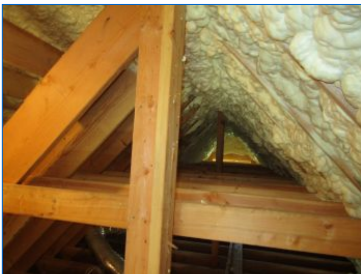
Vertical support of the roof ridge beam was noted.
