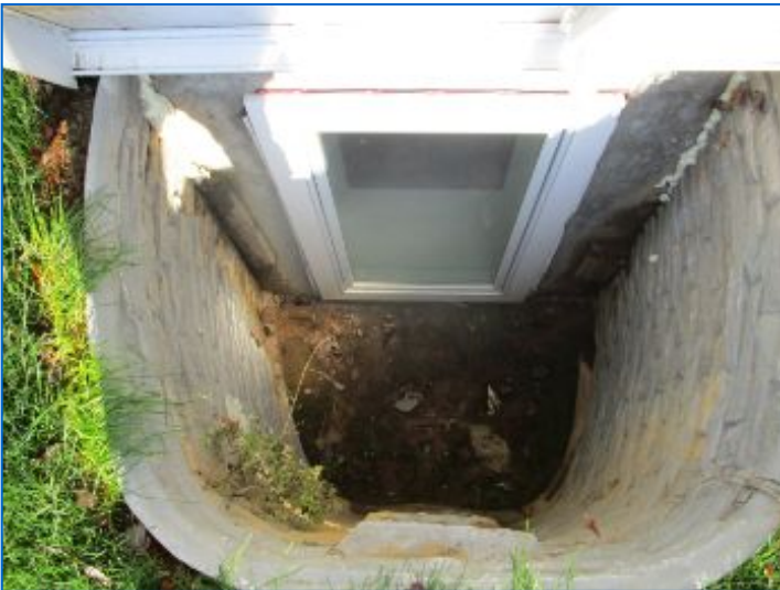
The basement had means of egress which complied with generally-accepted modern safety standards.
