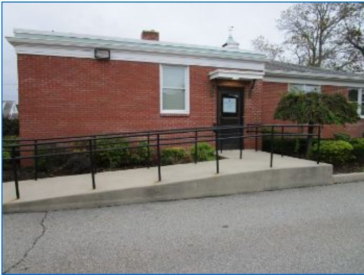
EXTERIOR East Exterior
