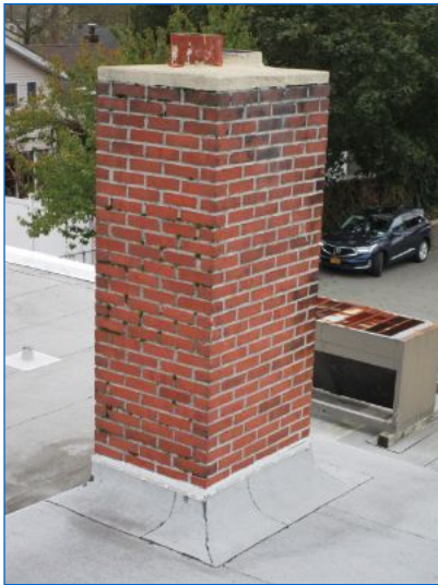
Double stack chimney noted.
