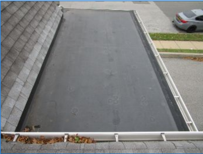
Canopy rubber membrane roof covering showed conditions consistent with 1 - 2 yr old materials.
