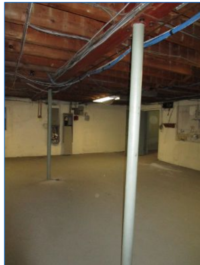
Main Floor Structure: Steel girder supported by steel lally columns and foundation walls, 2x10 Joists 16" O.C. (w/cross braces), T&G floor boards.
