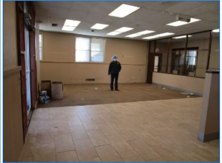
Interior Area 1 General
