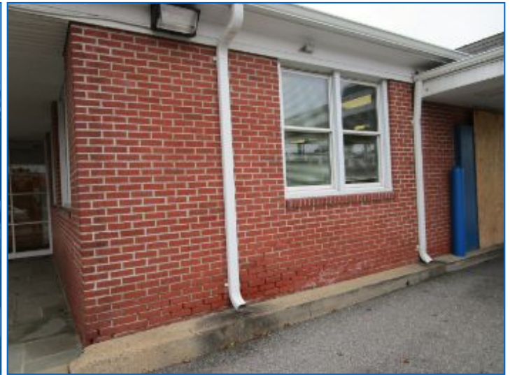
EXTERIOR West Exterior
