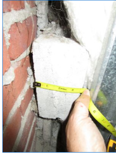
Exterior walls were built using 4" nominal concrete masonry units (CMU).
