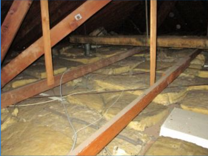
The inspector observed no significant deficiencies in the condition of the thermal insulation at the time of the inspection.
