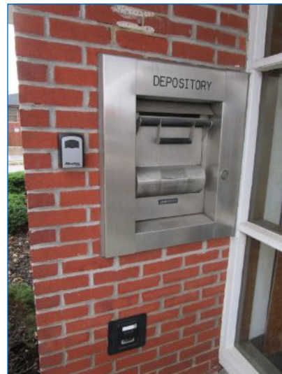
Exterior bank related equipment and components noted at front.
