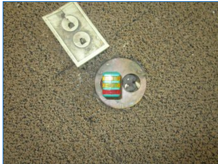
Floor area had a framed/raised floor system with floor recessed and surface mounted electrical/telecom receptacles installed.
