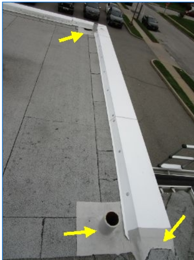
Recent roof repairs noted around roof penetration/flashings.
