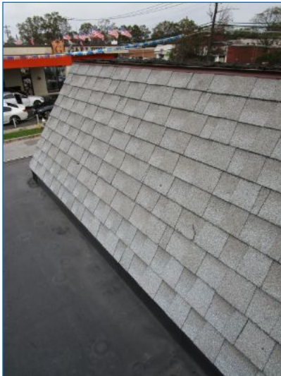
Roof over bank pneumatic tube conveyor consisted of architectural shingles, metal cap flashing and asphalt roll roofing.
