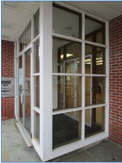
Front doors and vestibule included aluminum frame doors and wood constructed vestibule enclosure.
