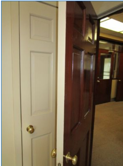
The building had mostly Solid wood panel interior doors.
