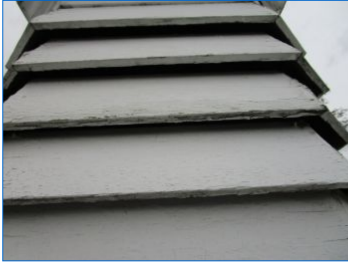
Apparent screen behind louvers.
