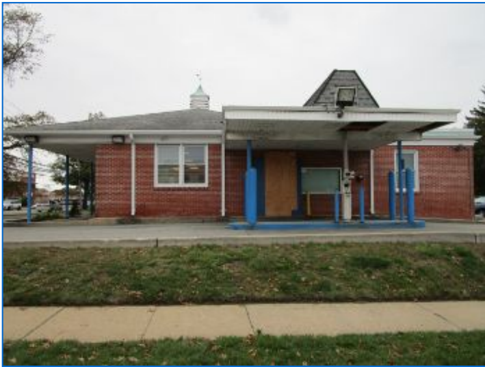
EXTERIOR West Exterior
