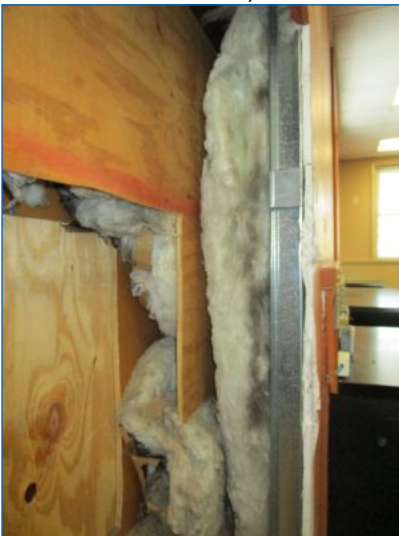
Walls: 2x4 metal studs (exterior walls insulated).
