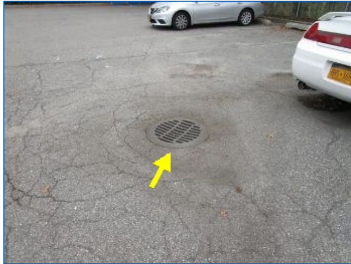
Driveway/parking lot was equipped with two visible drainage wells; SW drainage well.
