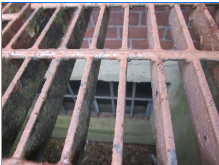
WINDOWS (Exterior) Basement Windows (Exterior)
