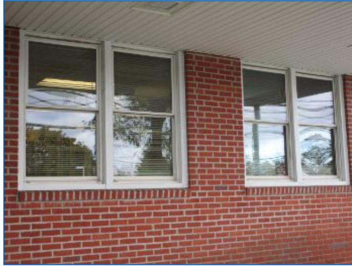
Main floor windows were Vinyl frame, Double-pane (insulated), Double hung windows.
