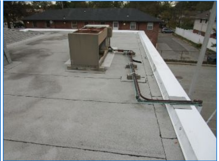
Rear flat roof.
