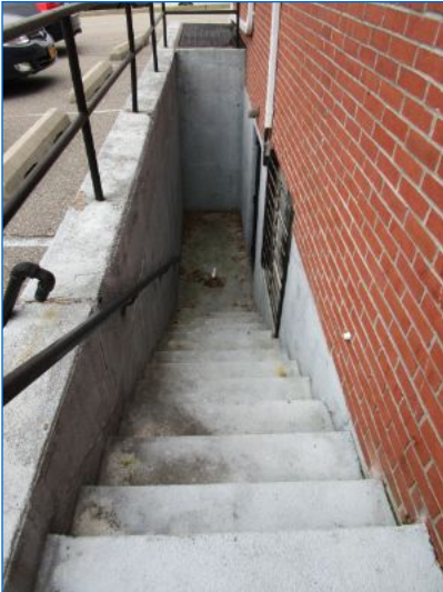
Exterior steps to basement. No system safety or function concerns noted at time of inspection.
