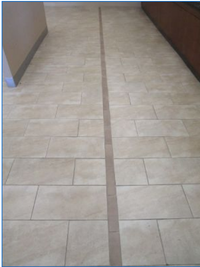
Porcelain tile floor noted.
