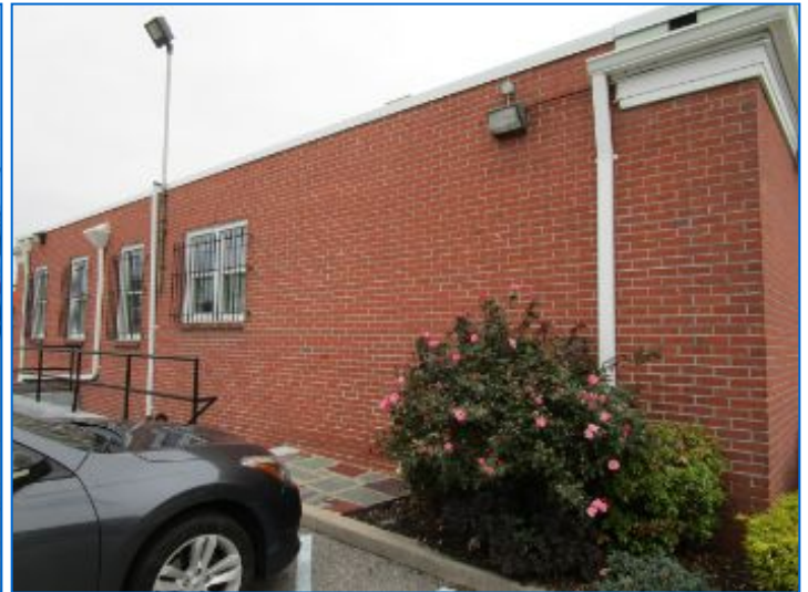
EXTERIOR South Exterior
