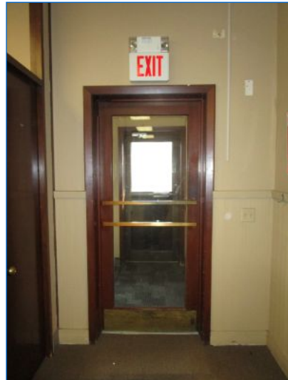
East vestibule; to handicap ramp.
