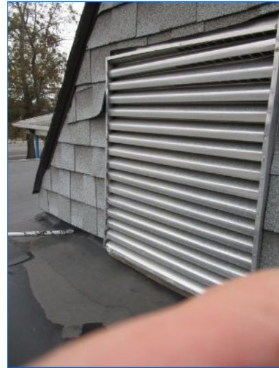
Gable-end louver vents noted for roof system ventilation.
