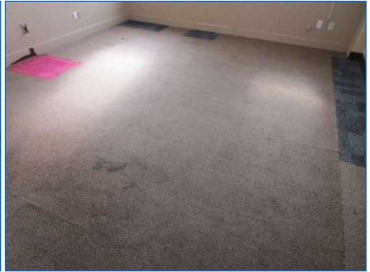
Carpeted floor noted.
