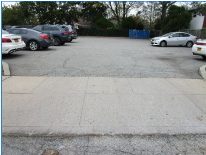
Driveway/Parking: Asphalt noted; Concrete aprons noted.
