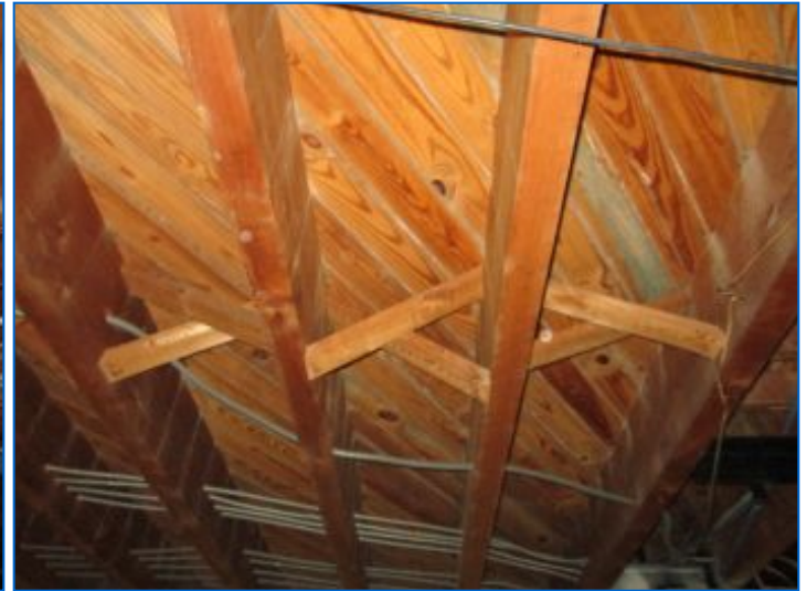
Main Floor Structure: Steel girder supported by steel lally columns and foundation walls, 2x10 Joists 16" O.C. (w/cross braces), T&G floor boards.
