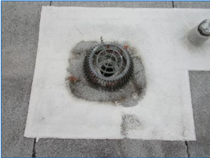
Roof drain appeared clear at flat roof.
