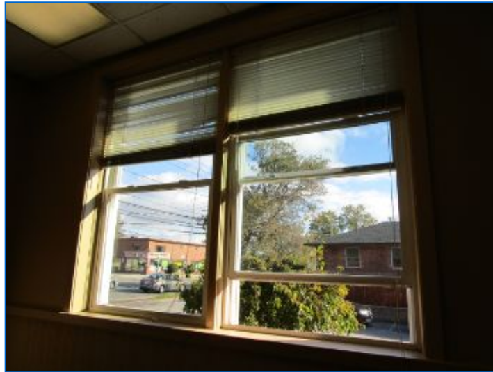
A representative number of window on the main levels were tested. All were operable when tested.
