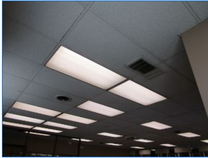
Acoustical tile w/grid ceilings noted.
