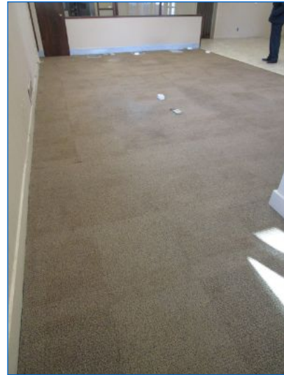
Carpeted floor noted. Floor area had a framed/raised floor system with floor recessed and surface mounted electrical/telecom receptacles installed.
