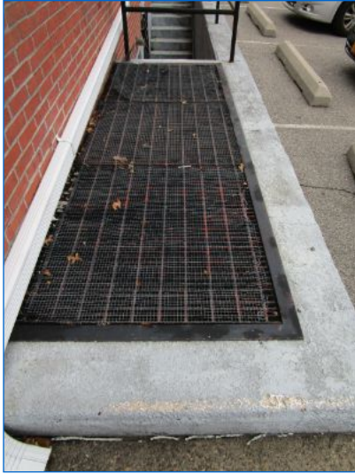
Concrete window wells with steel grating noted at east and south sides. No system safety or function concerns noted at time of inspection.
