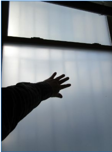
Teller Admin: Frosted windows with burglar bars noted.
