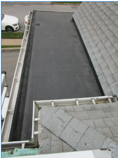
Roof covering consisted of a combination of Architectural asphalt shingles and Rubber membrane (flat roof).
