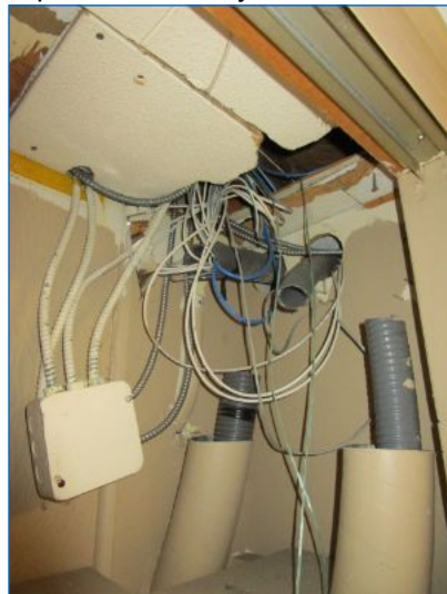
Cafeteria: Former telecom closet.
