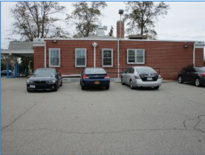
EXTERIOR South Exterior
