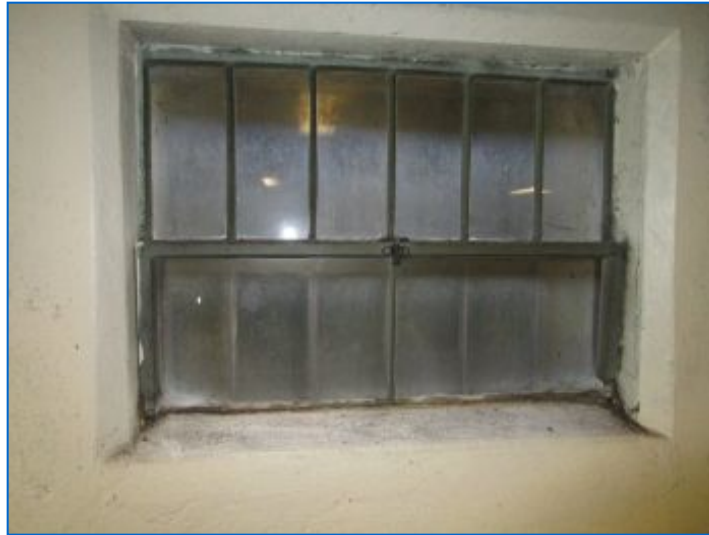
Basement windows were Steel frame, hopper style, Single-pane (non-insulated) windows.
