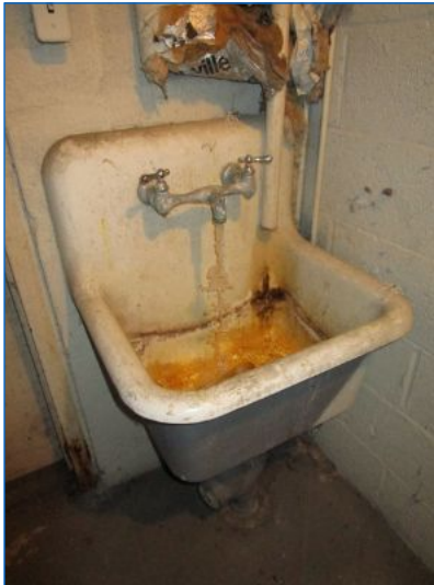
Equipment Room: Old service sink had functional flow and drainage.
