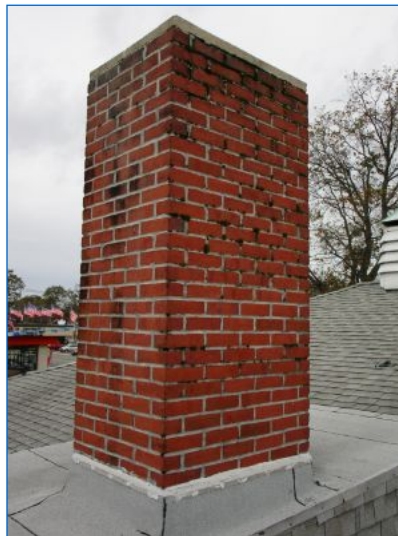
The Inspector observed no deficiencies in the condition of the visible portions of the chimney structure.
