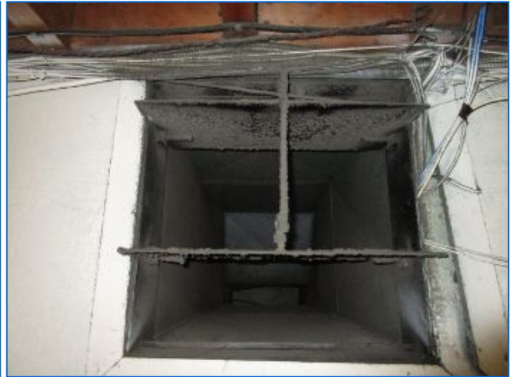
General Area: Duct appeared to be part of an old exhaust/ventilation system; defunct.
