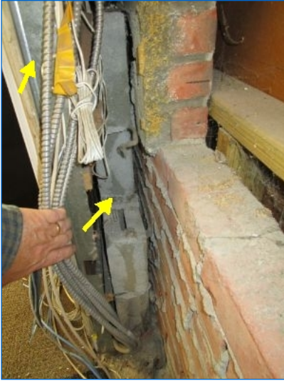
Exterior walls were built using 4" nominal concrete masonry units (CMU). Walls: 2x4 metal studs (exterior walls insulated).
