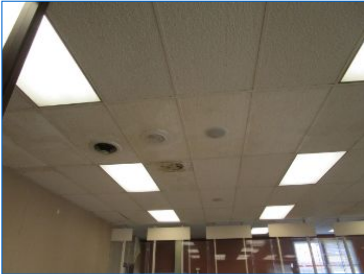
Ceiling: 2'x4' Acoustical tile w/grid and recessed light fixtures noted.
