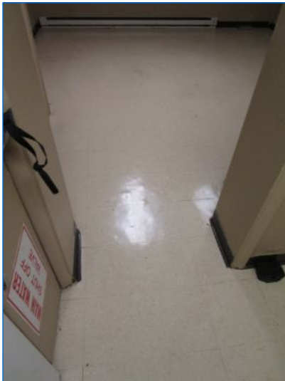
Cafeteria & Pantry: Floor covering was Vinyl Composition Tile (VCT)
