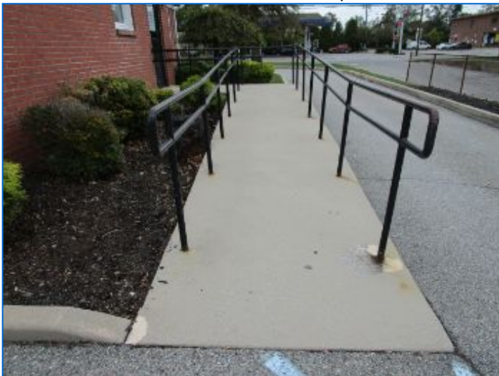
Concrete handicap ramp at east side entrance.
