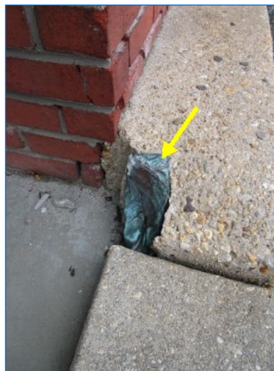
Original copper downspout connection to drywell at NW corner was terminated.
