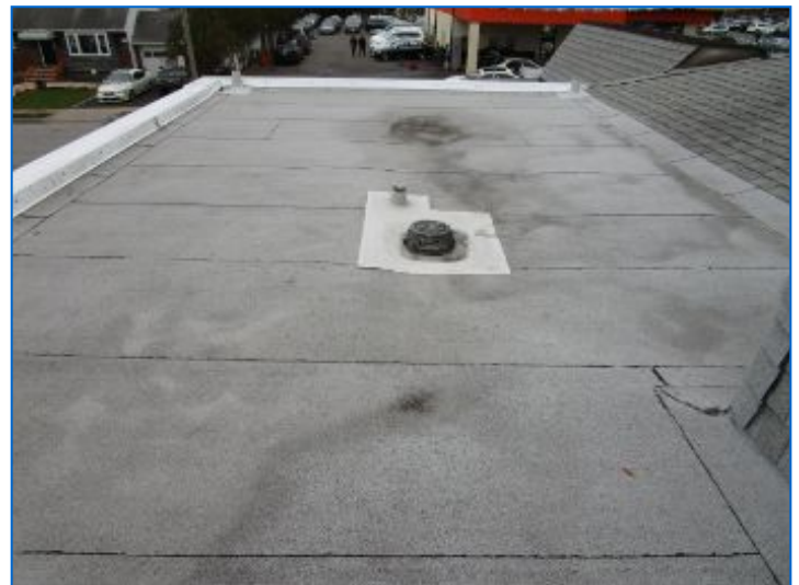
Asphalt roll roof covering showed conditions consistent with 15 yr old material.
