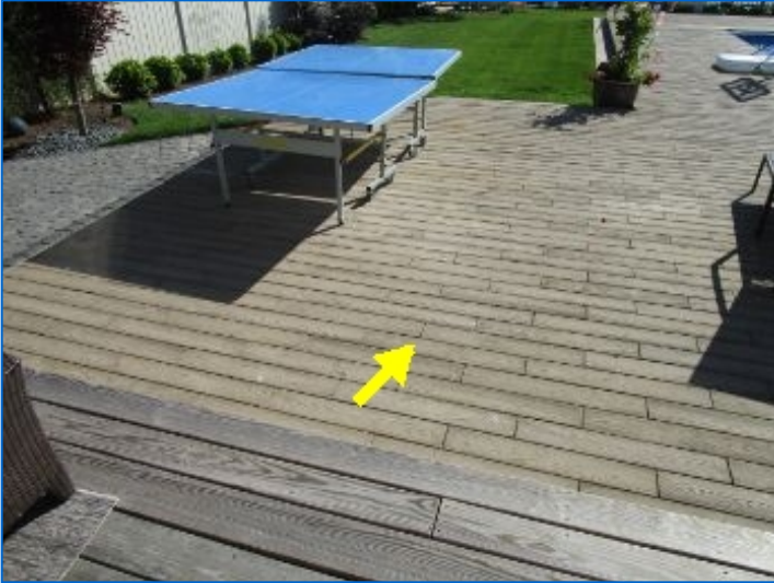
Concrete barnwood plank pavers noted at patio.
