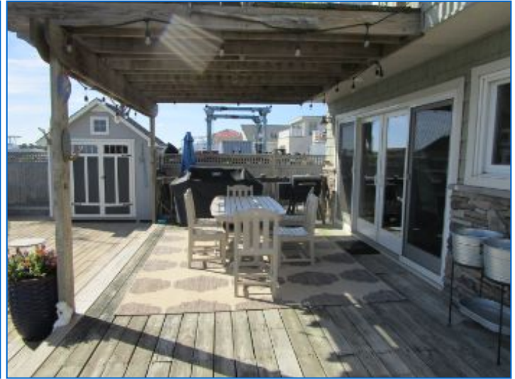
DECK AREA Deck General
