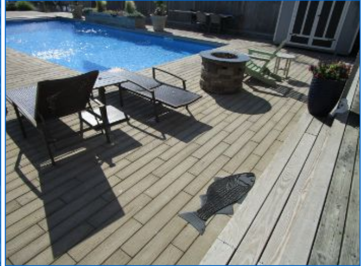
Concrete barnwood plank pavers noted at patio.
