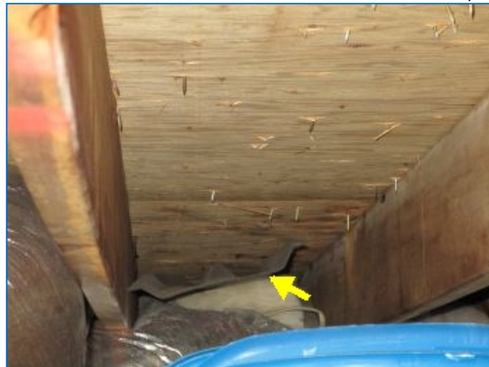
Some insulation baffles noted to facilitate under eave soffit venting.
