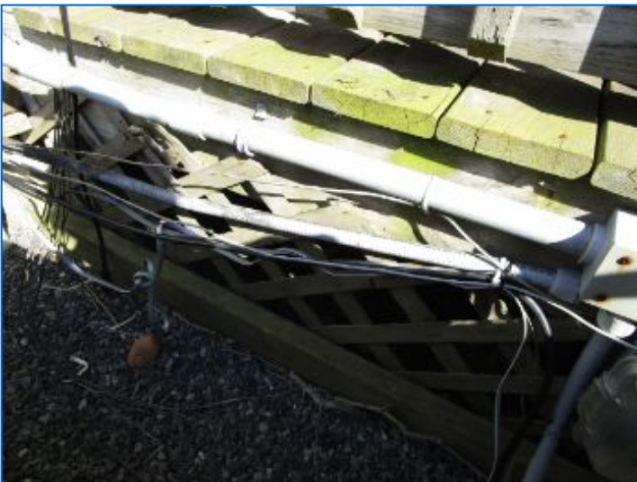
Limited review of deck foundation due to limited or no access below.
