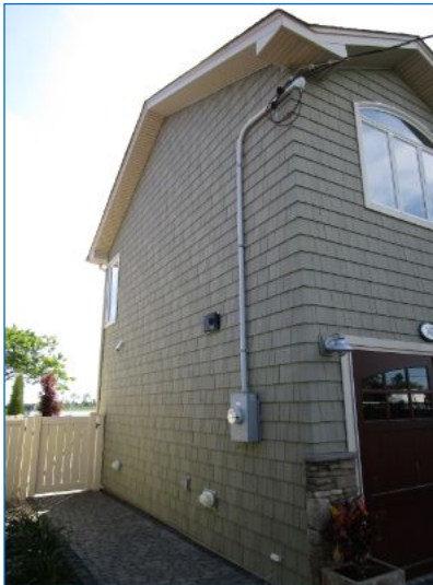
EXTERIOR South Exterior
