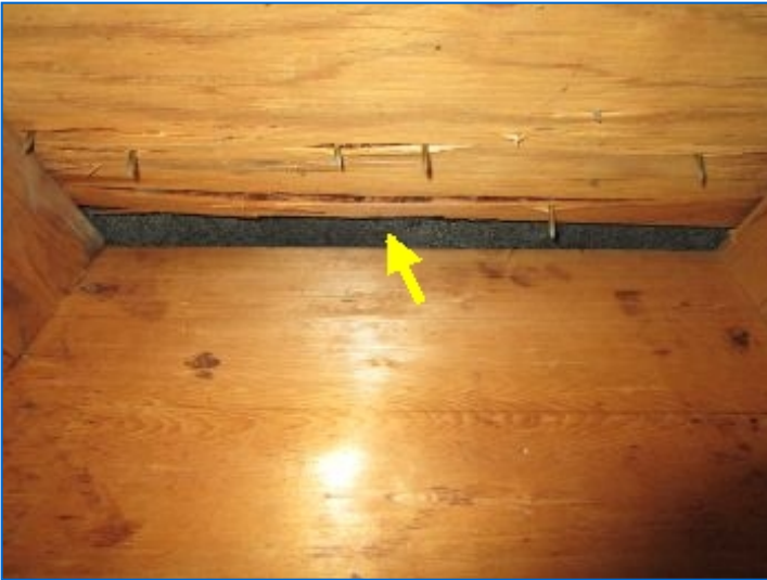
Ridge exhaust venting noted
