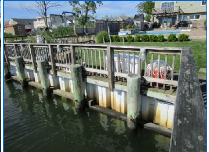
Bulkhead appeared to be well constructed, however not all structural components of the bulkhead system are visible. Suggest acquiring drawings and specs as available for further review by a bulkhead specialist.
