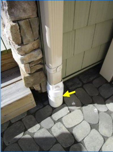
Downspouts connect to underground drainage system/s; drywell/s.
