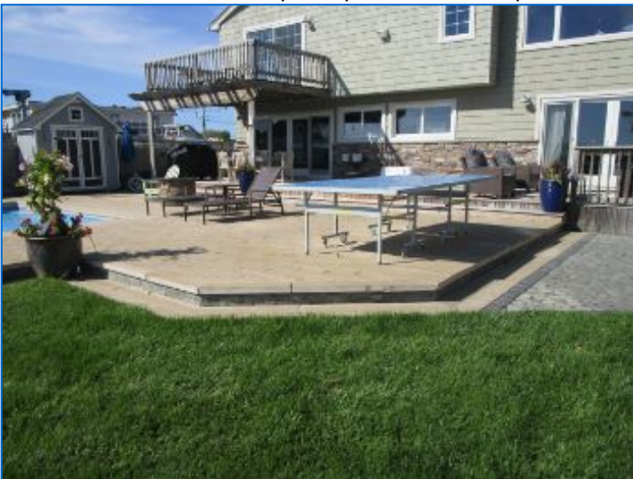
Patio appeared in satisfactory and functional condition.
