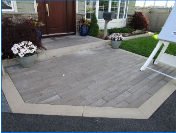
Concrete barnwood plank paver Steps and Landing noted at Front entrance.
