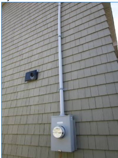
Overhead electrical service drop and riser showed no system safety or function concerns at time of inspection.
