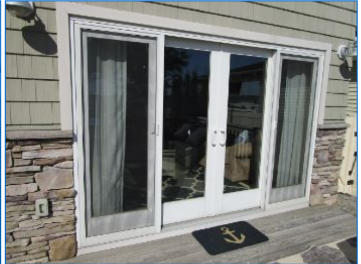
Rear doors to den.
