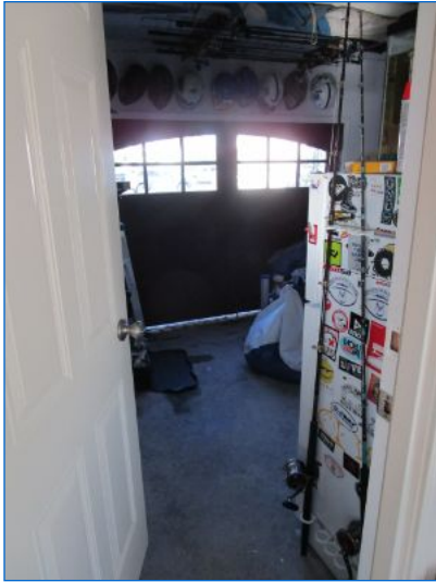
GARAGE General Conditions
