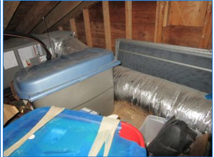
Not all areas of the attic were accessible due to heavy storage of personal items.
