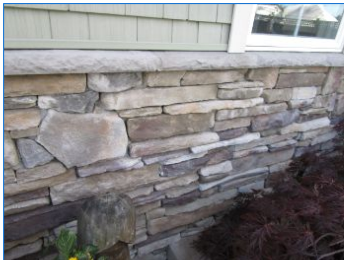
Stone veneer appeared to be in satisfactory condition - In normal condition for its age.
