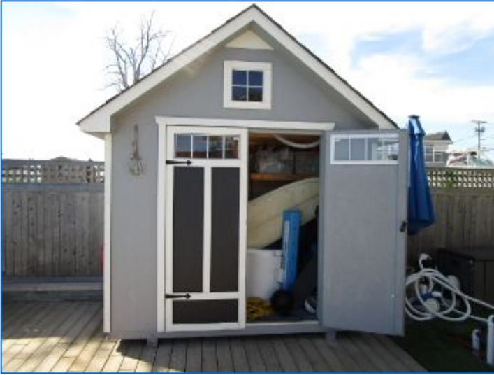
No major defects noted for visible structure of the shed - in normal condition for its age.
