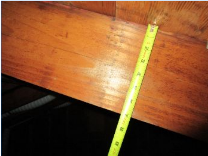
Main Roof Structure: 2x8 Rafters 16" O.C., 2x10 ridge beam, Plywood roof boards.
