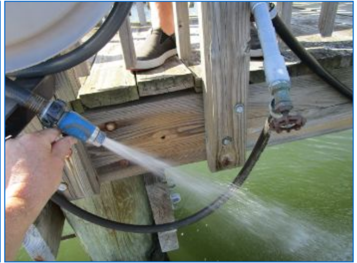
Hose bibs were operable at time of inspection.
