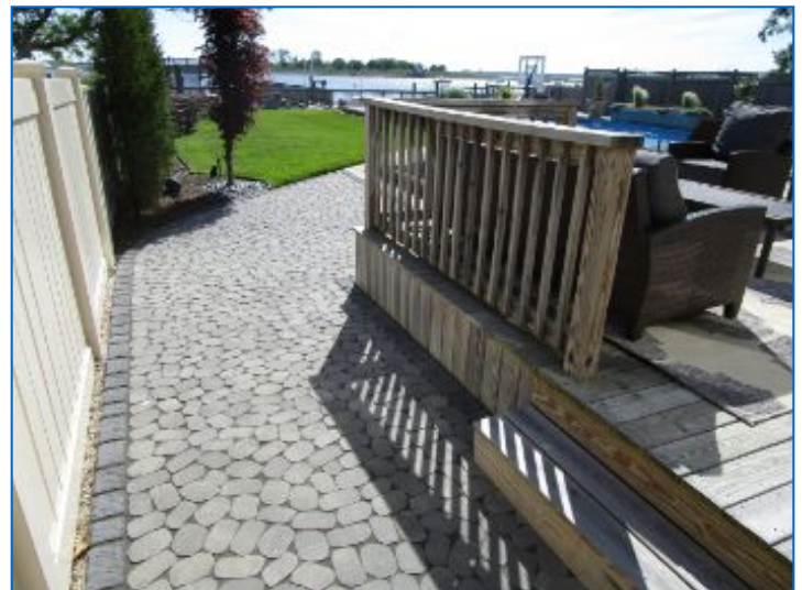
GROUNDS Sidewalk & Walkway
