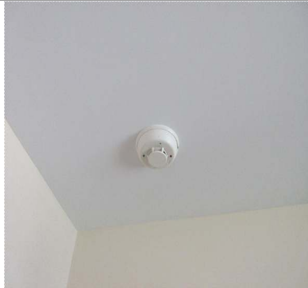
IMG_0276.JPG Maintain functioning smoke and carbon monoxide detectors. Detectors are generally reliable for up to five years.
