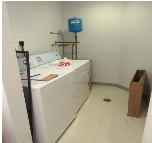
IMG_0285.JPG Laundry/utility room with floor drain..
