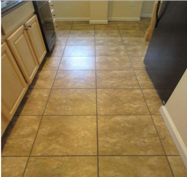
IMG_0264.JPG Kitchen floor in good condition.
