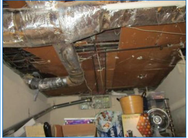
Ceiling conditions in southwest room in basement.
