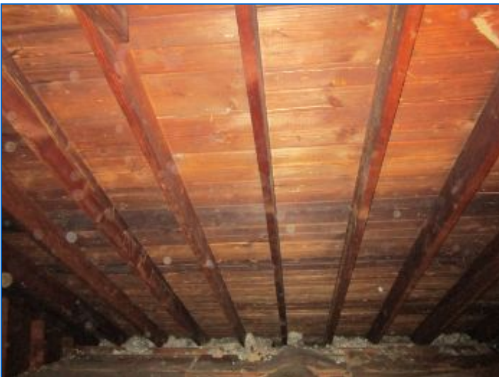
Visible areas of the roof structure appeared satisfactory.
