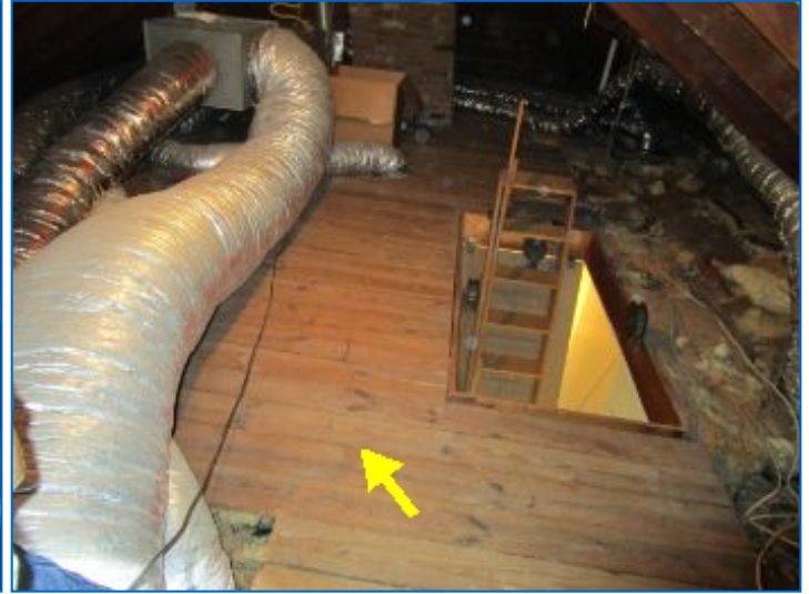
Attic floor Partially covered with permanent floor boards.
