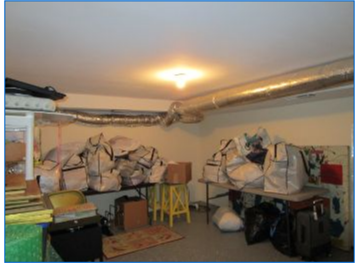
Northwest corner room.
