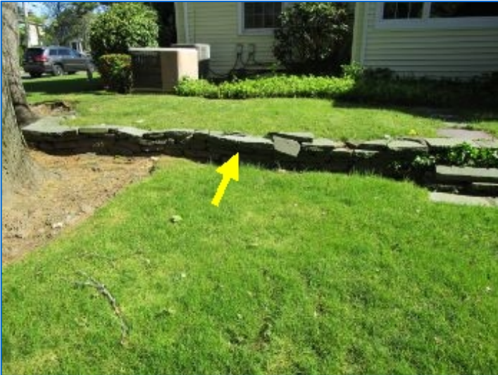
Stone retaining wall noted.
