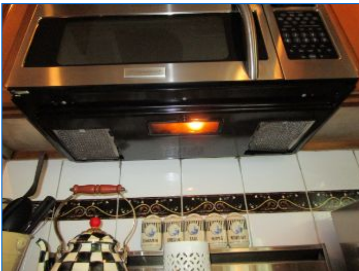
Microwave had an operable built-in Recirculating vent fan with grease filter and light.
