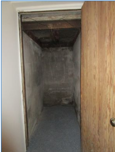
Basement extension under garage with steel access doors above.
