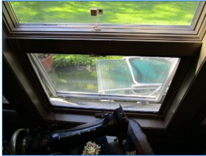
Wood framed awning windows noted in the Den.
