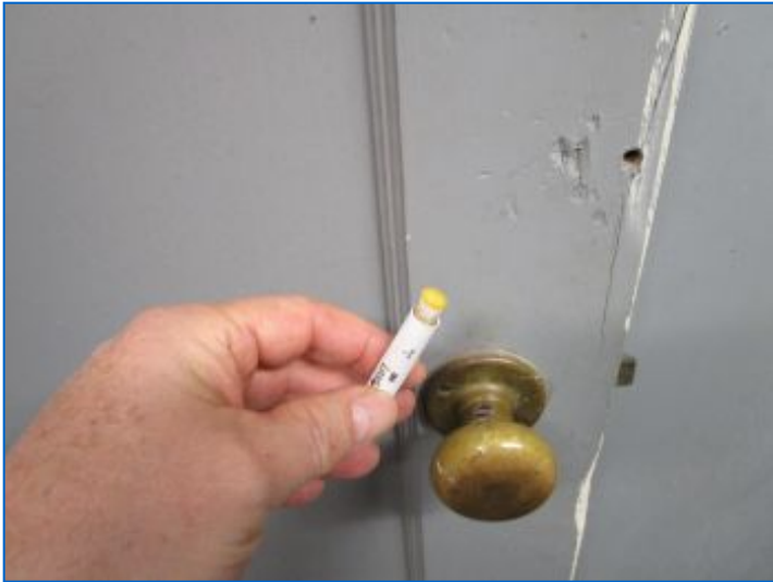
Testing for surface lead paint conducted in Basement; test results were negative.
