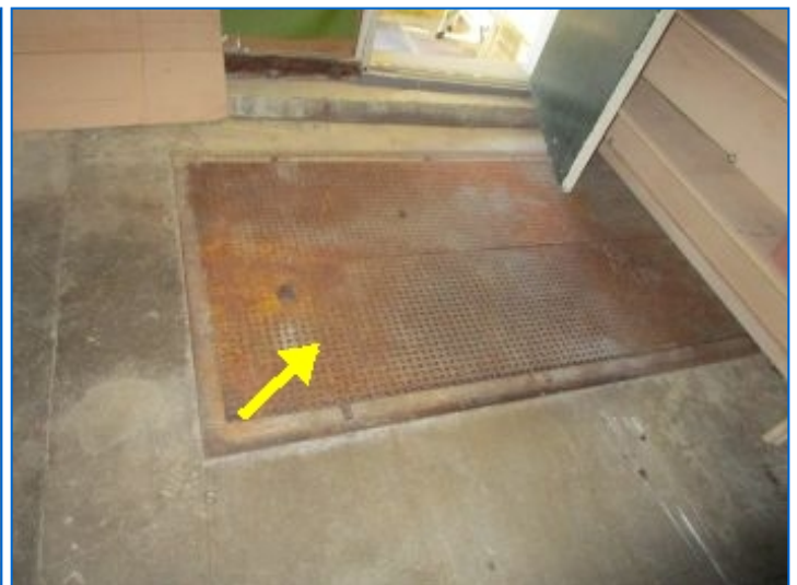
Steel plate floor hatch in garage to basement.
