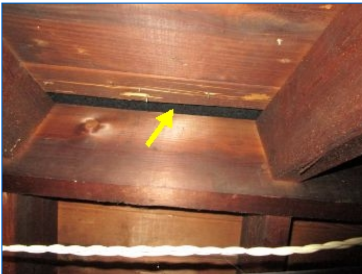
Ridge exhaust venting noted
