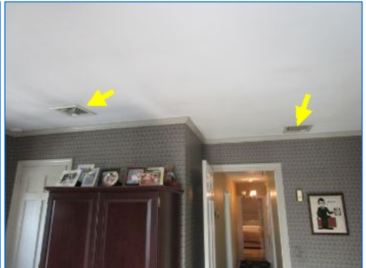
Office heating is via ducted HVAC#2 system
