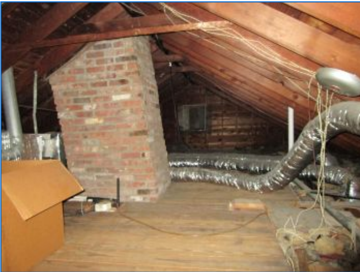
ATTIC Attic General
