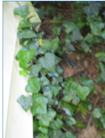
Ivy can grow aggressively; attracts insects and can damage siding and trim; suggest removing ivy that is in close proximity to the home.
