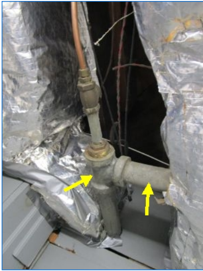
Galvanized DWV pipe noted.
