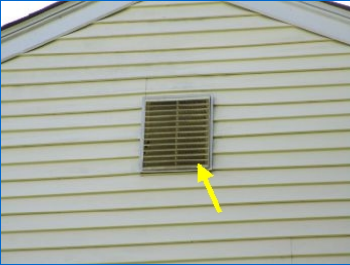
Gable-end louver vent(s) noted for attic ventilation.
