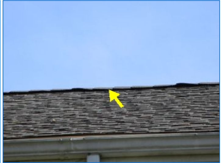
Upper roof ridge exhaust venting noted for attic ventilation.
