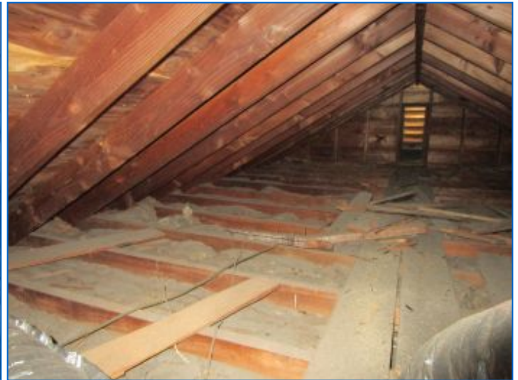
Attic space over garage.
