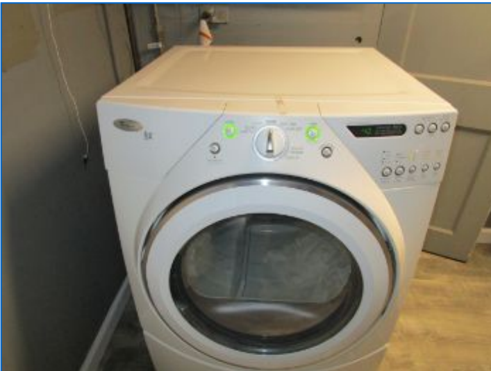
Gas dryer was operable. Estimated age of the dryer is 5+ yrs.
