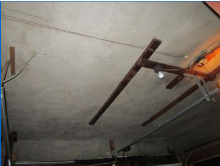
Lightweight concrete wall and ceiling finish noted.
