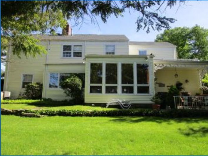
EXTERIOR North Exterior
