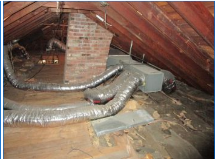
ATTIC Attic General
