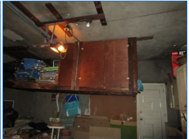
Limited review due to shelving/cabinets and stored items.
