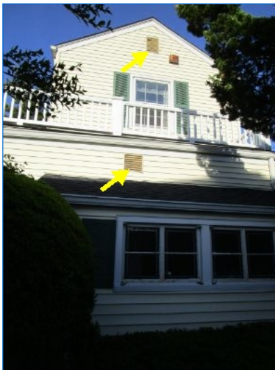
Gable-end louver vent(s) noted for attic ventilation at west exposure.
