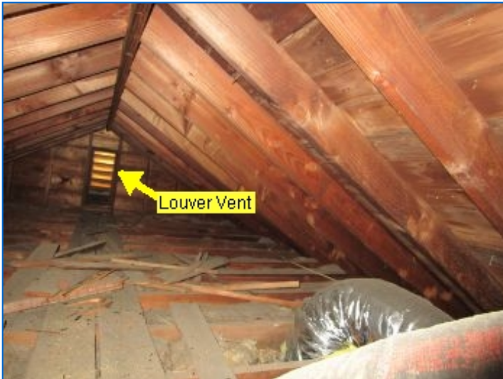
Attic space over garage.
