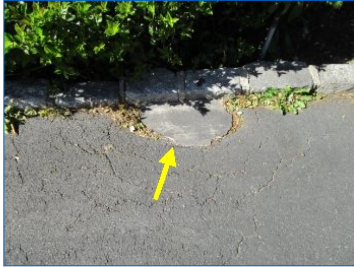
Patch repair noted in driveway.
