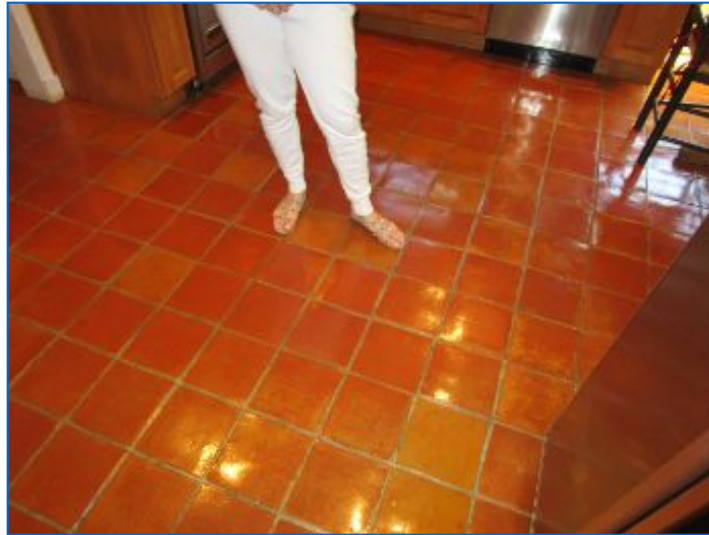
Ceramic/Porcelain tile flooring noted. No defects noted.
