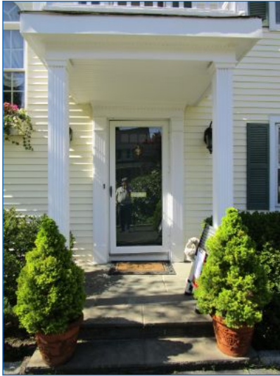
Front door bell operated normally when tested.
