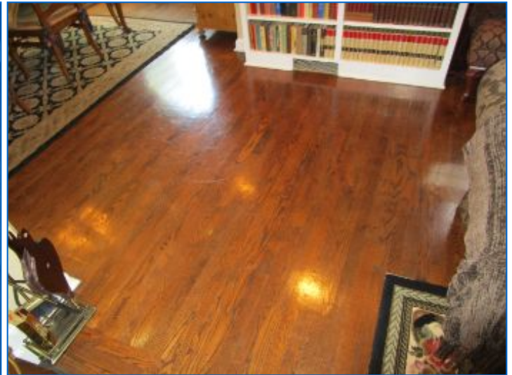
Solid hardwood floor noted.
