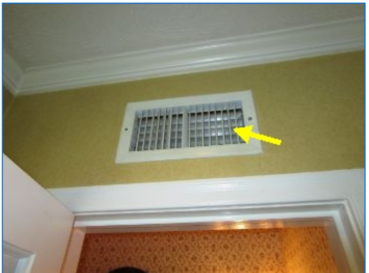
Transfer grille noted over bathroom door.
