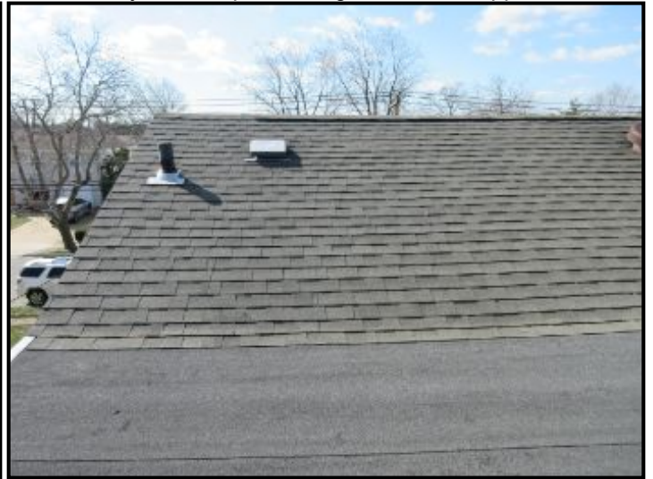
Rear roof looking south.
