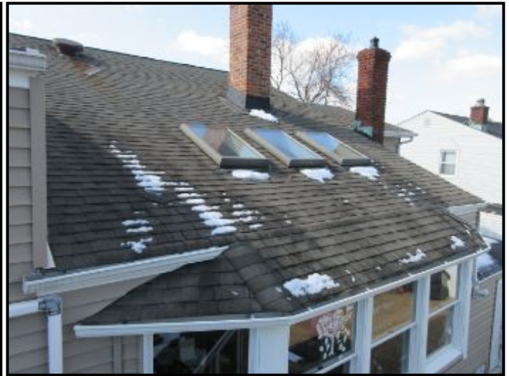
Asphalt shingles noted.
