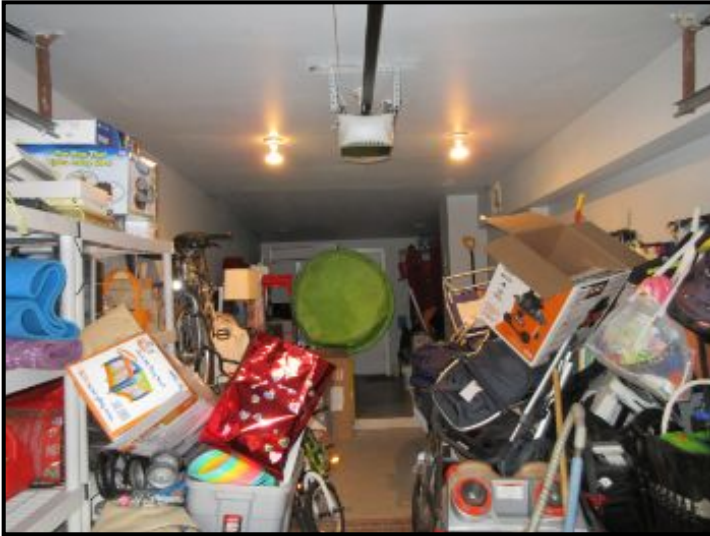
Garage walls and ceiling finished in drywall. Condition was filled with stored items.
