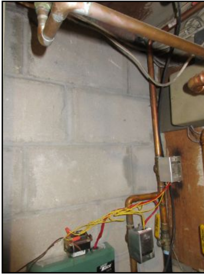
Foundation: Concrete Block also noted
