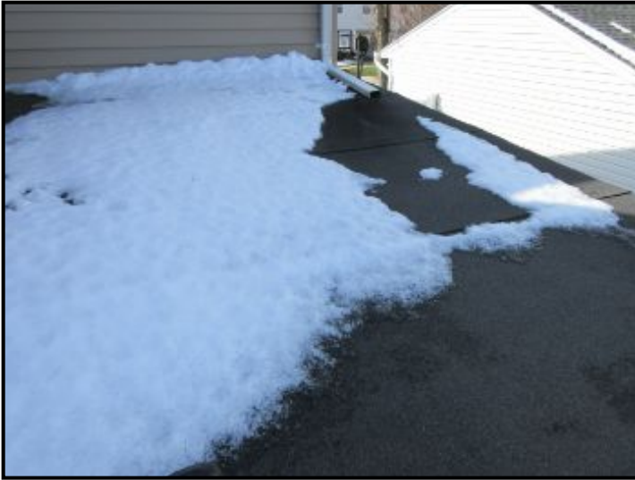
Asphalt rolled roofing noted.
