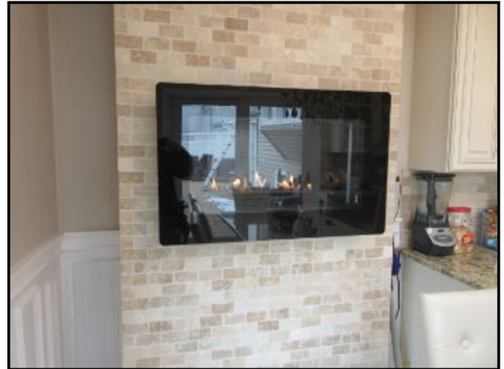
Kitchen nook fireplace noted. Gas fireplace operable.
