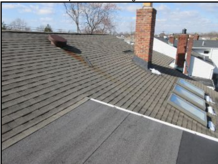
Roof looking west.
