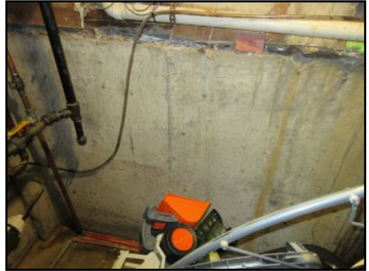
Foundation: Poured Concrete (w/stucco veneer).
