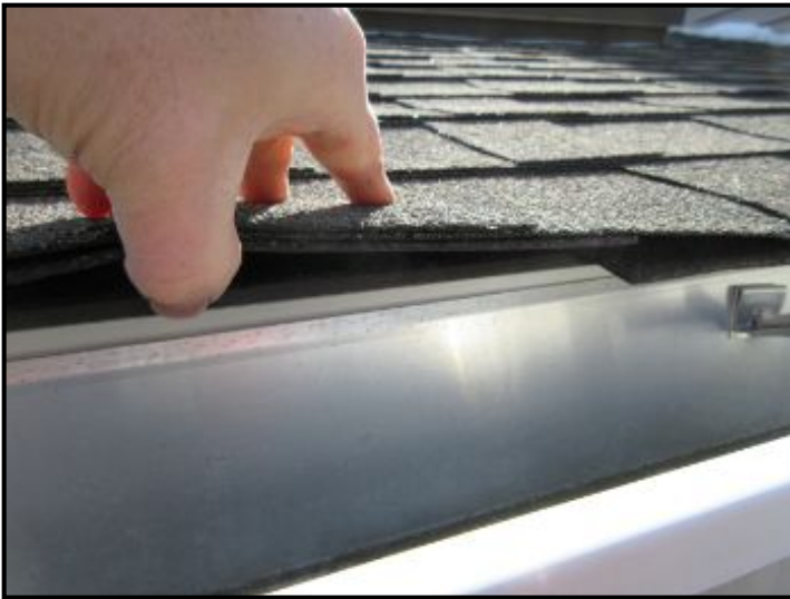
One layer of asphalt shingles noted at roof of kitchen addition.
