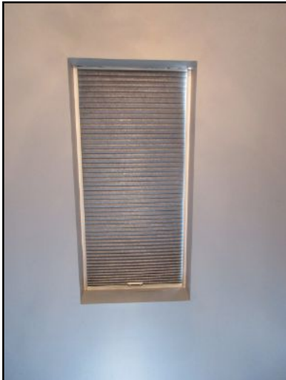
Master bedroom skylight appeared serviceable.
