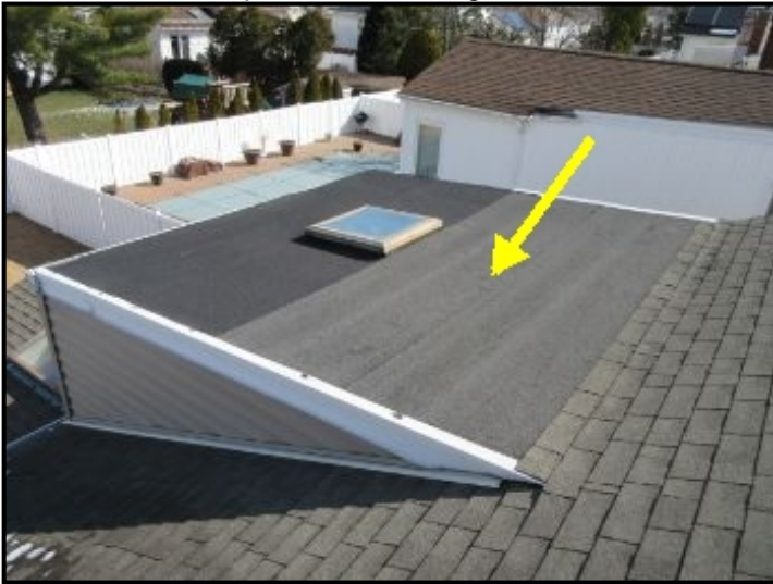
Asphalt rolled roofing noted.
