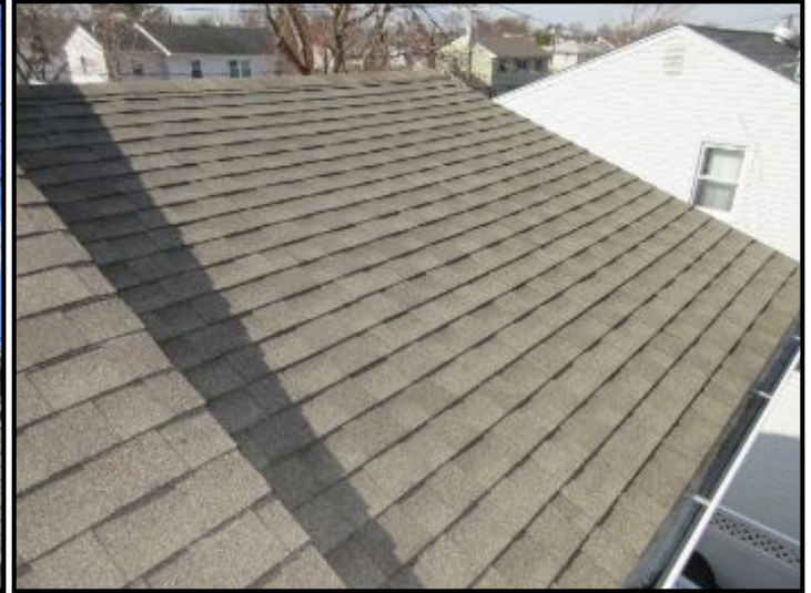
Top asphalt roof covering appeared to be approximately 6 yrs old.
