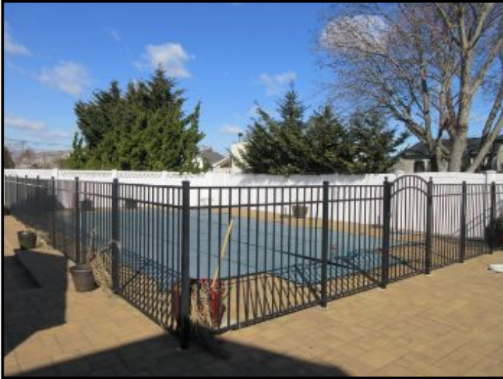
Pool area aluminum fencing in serviceable condition.
