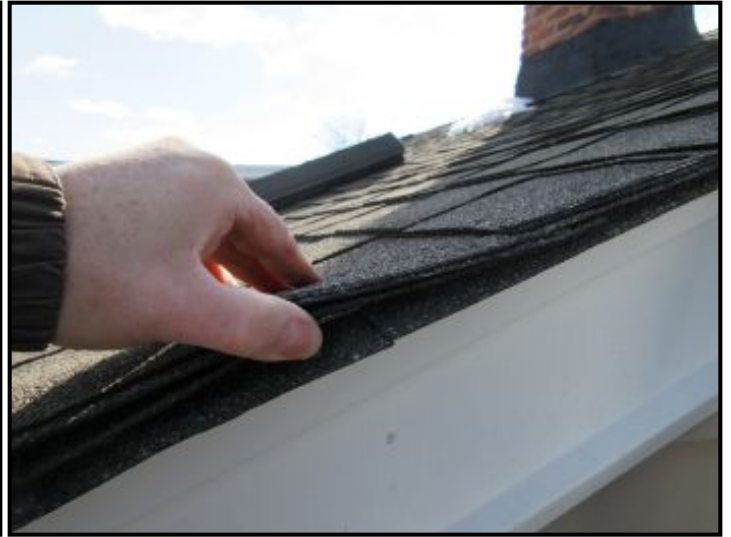
Two layers of asphalt shingles noted at upper roof.
