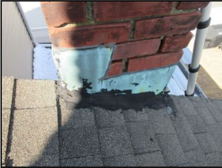
Copper flashing visible around chimney.
