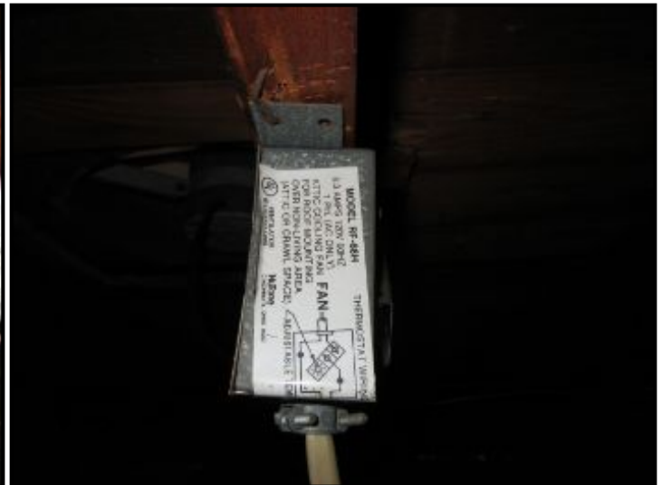
Thermostat functionality is questionable for Power Ventilator
