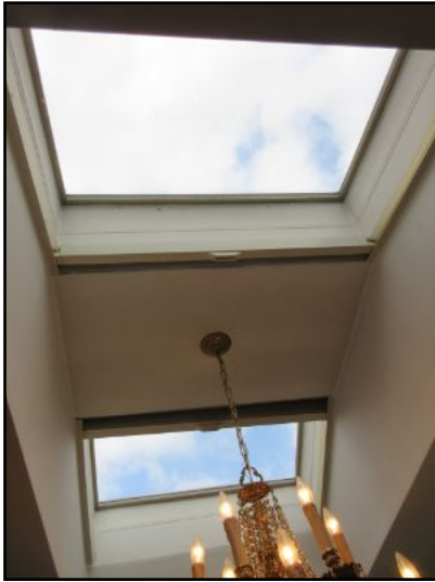
Kitchen skylights appeared serviceable with only minor cosmetic updates needed.
