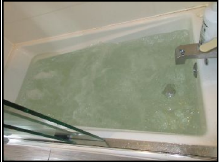
Whirlpool pump was operable.
