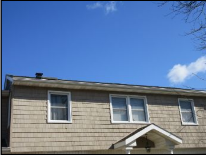
Roof ridge beam appeared straight and even.
