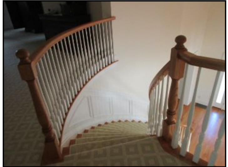
Main stairs and hand railing in good condition.
