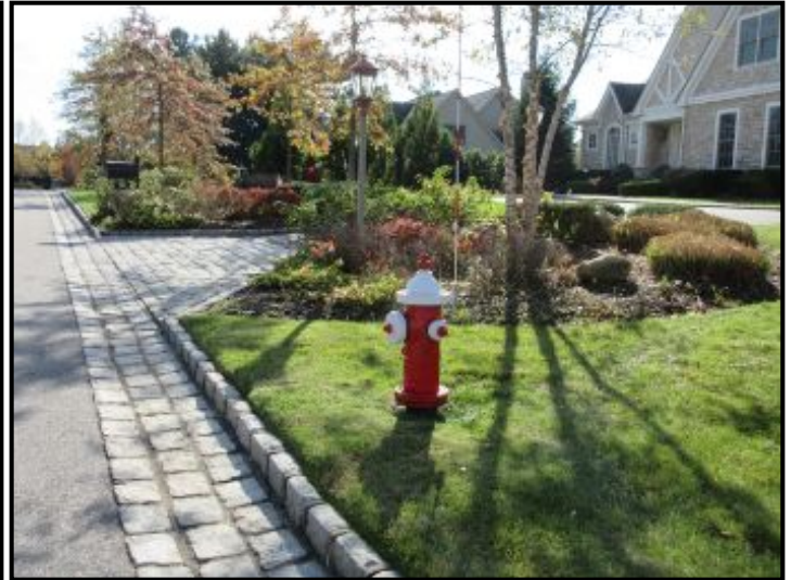
Belgium block curb and driveway aprons in good condition.
