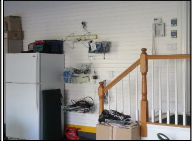
Garage wall hanging system noted.
