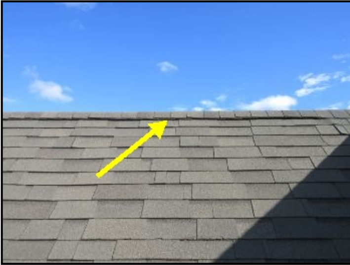
Ridge vent noted for attic ventilation.
