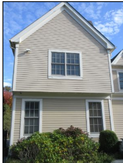
Rear left-side bay exterior.
