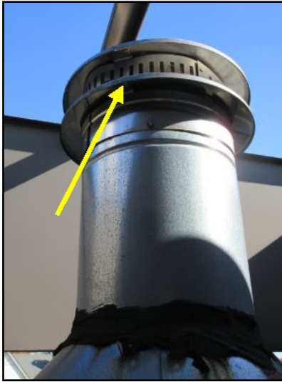
Chimney caps with spark arrestor noted.
