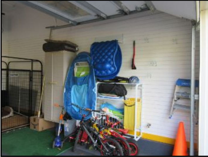
Garage wall hanging system noted.
