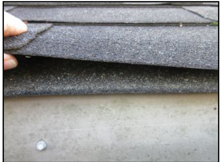
Ice shield observed beneath lower roof shingles.
