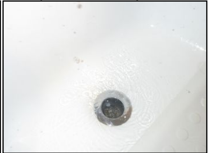
Tub stopper missing.
