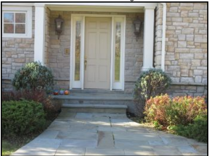
Bluestone (cleft cut) walkways.
