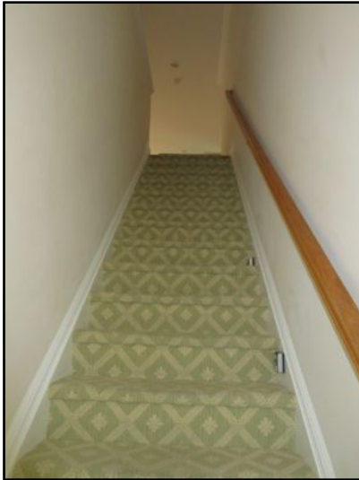
Service stairs and hand rail in good condition.
