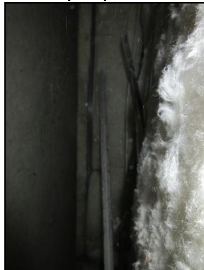
Accessible wall cavities were dry; no musty odor.
