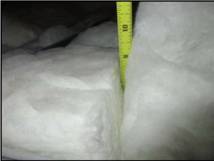
Insulation averages about 8-10 inches in depth.; Adequate.
