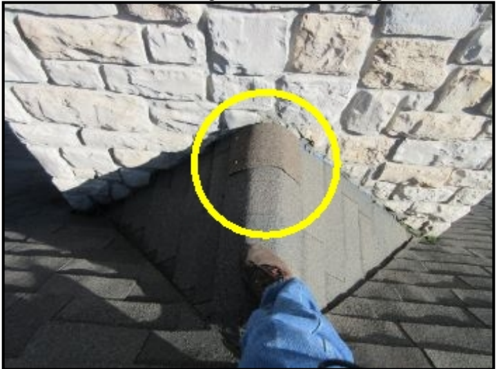
Shingle repair noted at chimney crickets.
