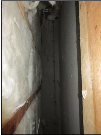
South wall cavity was dry; no musty odor.
