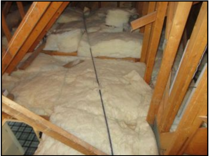
Fiberglass batts with kraft paper facing noted.
