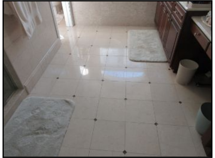
Marble tiled floor in good condition
