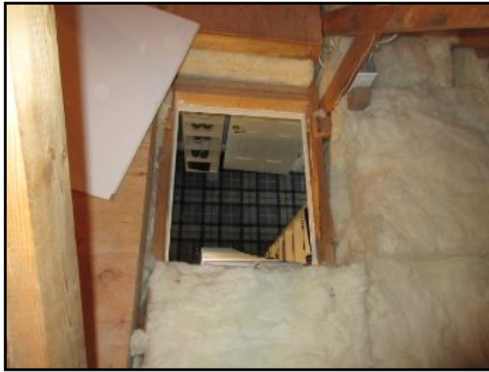
Attic accessed via Scuttle hole located in Boy's bedroom.
