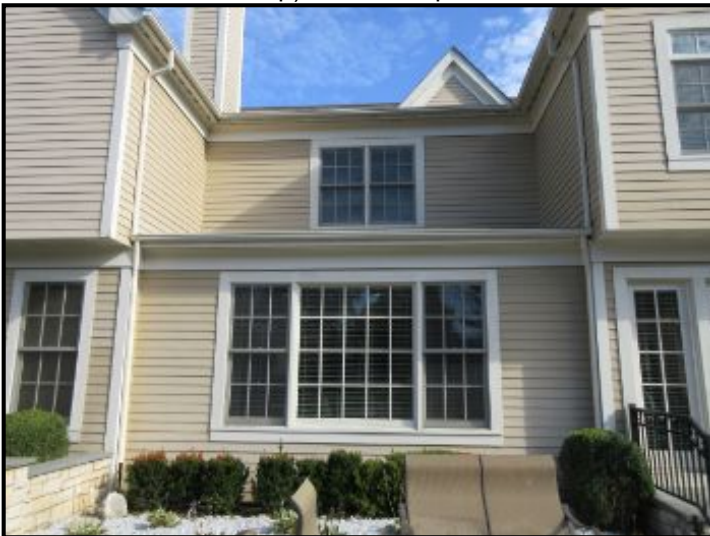
Rear center bay exterior.
