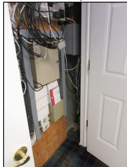
Checking south wall cavity conditions at electrical closet.
