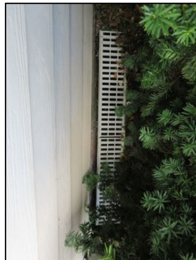
French drains observed in planting beds along the rear exterior wall.
