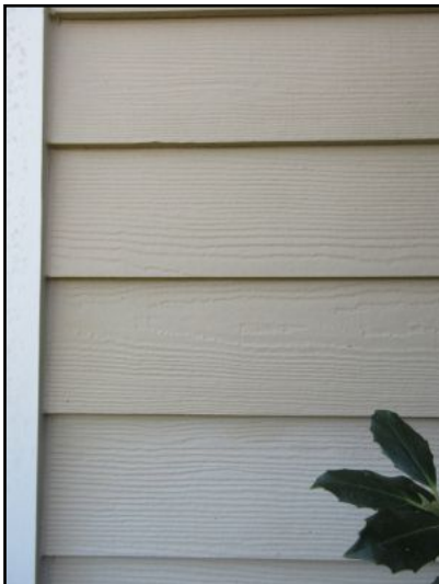
Fiber-cement siding noted.
