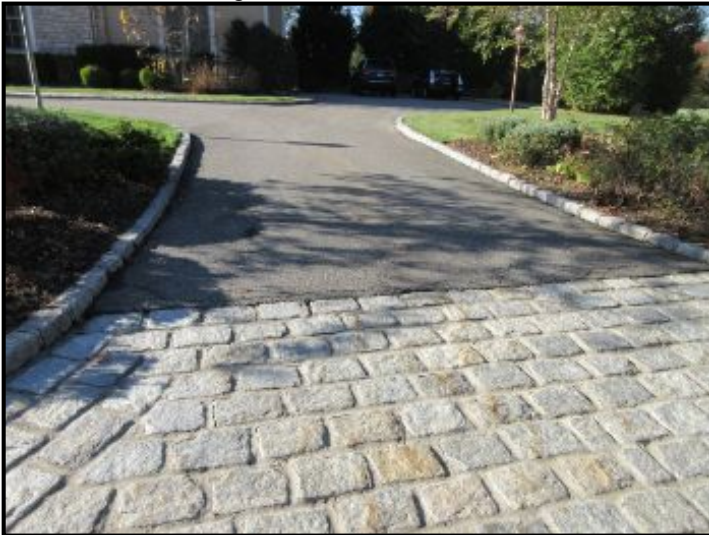
Belgium block driveway aprons in good condition.
