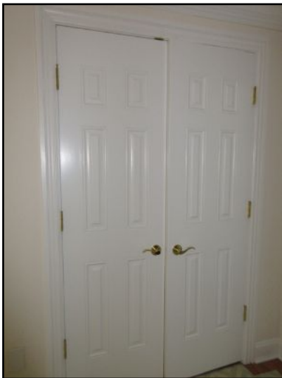
2nd floor double door closet.
