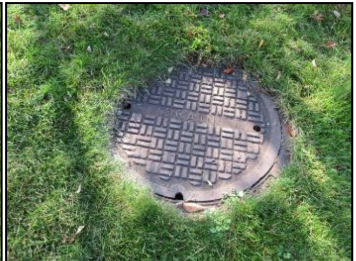
Storm water drain access at front lawn.
